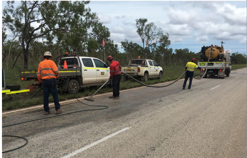
Figure 3: Spill clean-up efforts via pressure cleaner and industrial road sweeper at one of the spill locations.
