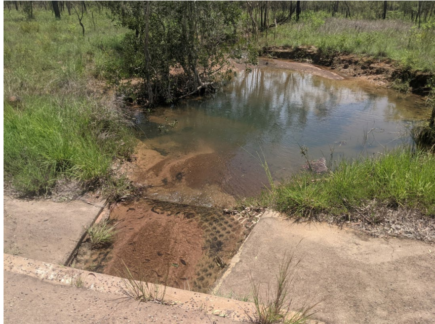
Figure 4: Site 1 – minor creek culvert observed next to spill location.
