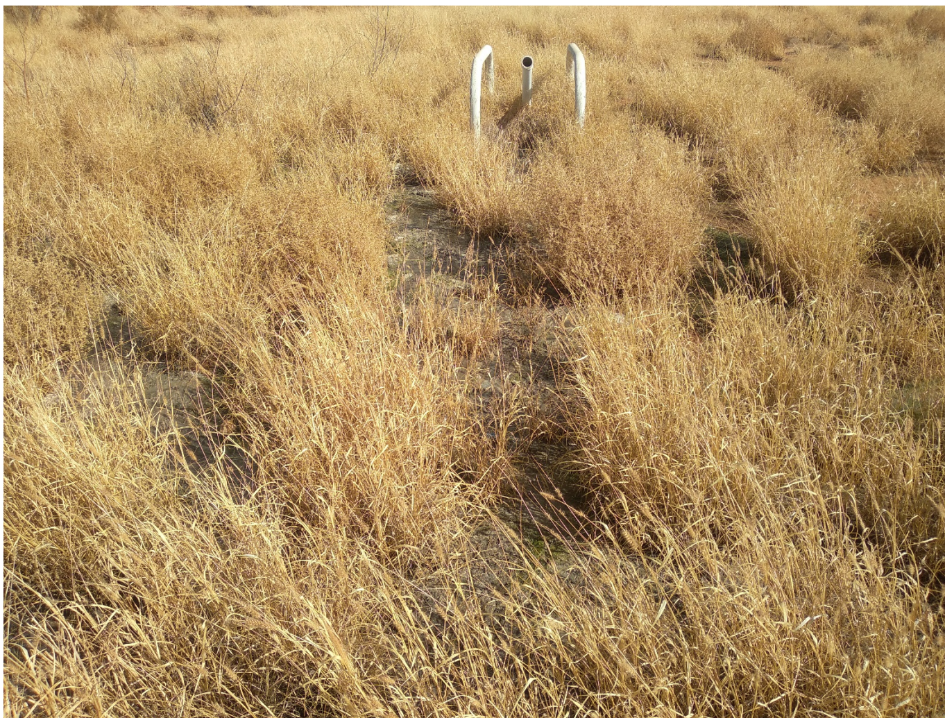
Photo 1 – Scour pipe and overflow area
