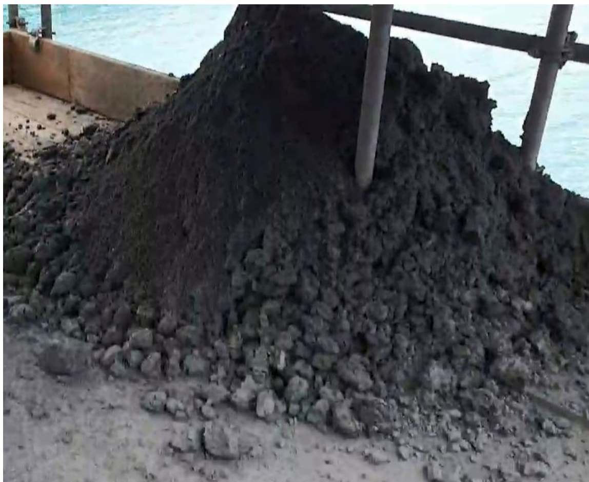
Figure 3: Build-up of material (manganese fines) on scaffold, located below the conveyor system. Some of the material has breached the walls of the scaffold and entered the ocean.
