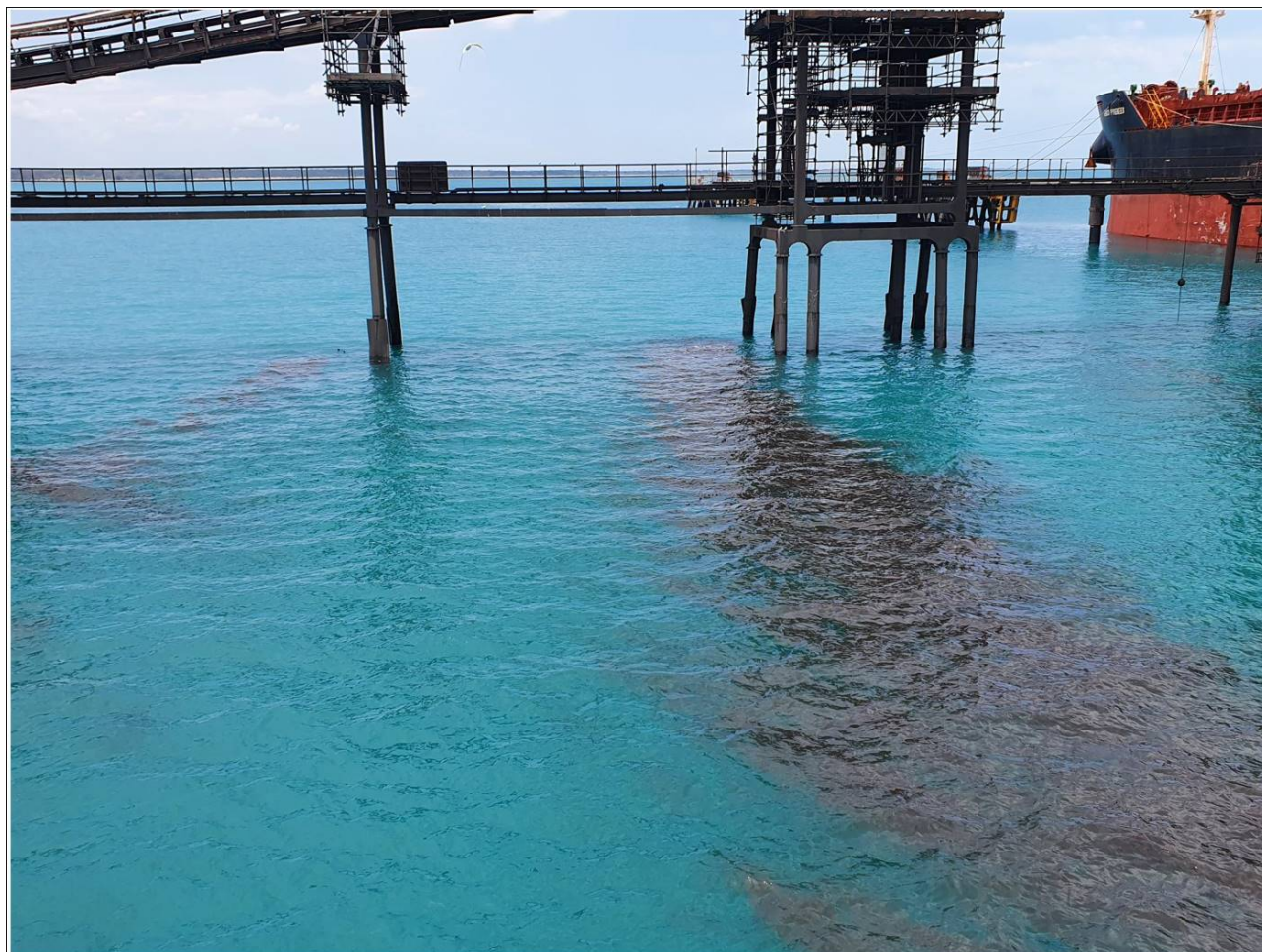
Figure 2: Manganese spillage and plume inside GEMCO's harbor facility (SPL382) – Photo taken 3rd October 2021.
