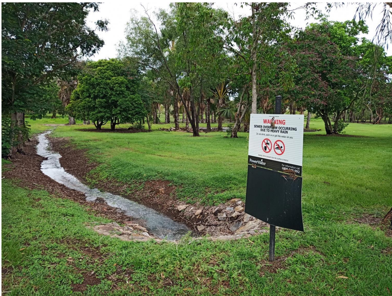
Appendix B – Photographs (Discharge point for SRV at 24 East Point Road, Fannie Bay, showing warning signage)
