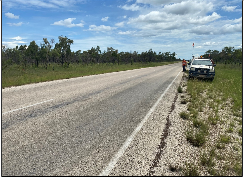
Figure 4: Site 2 – concentrate observed on road prior to clean-up efforts.
