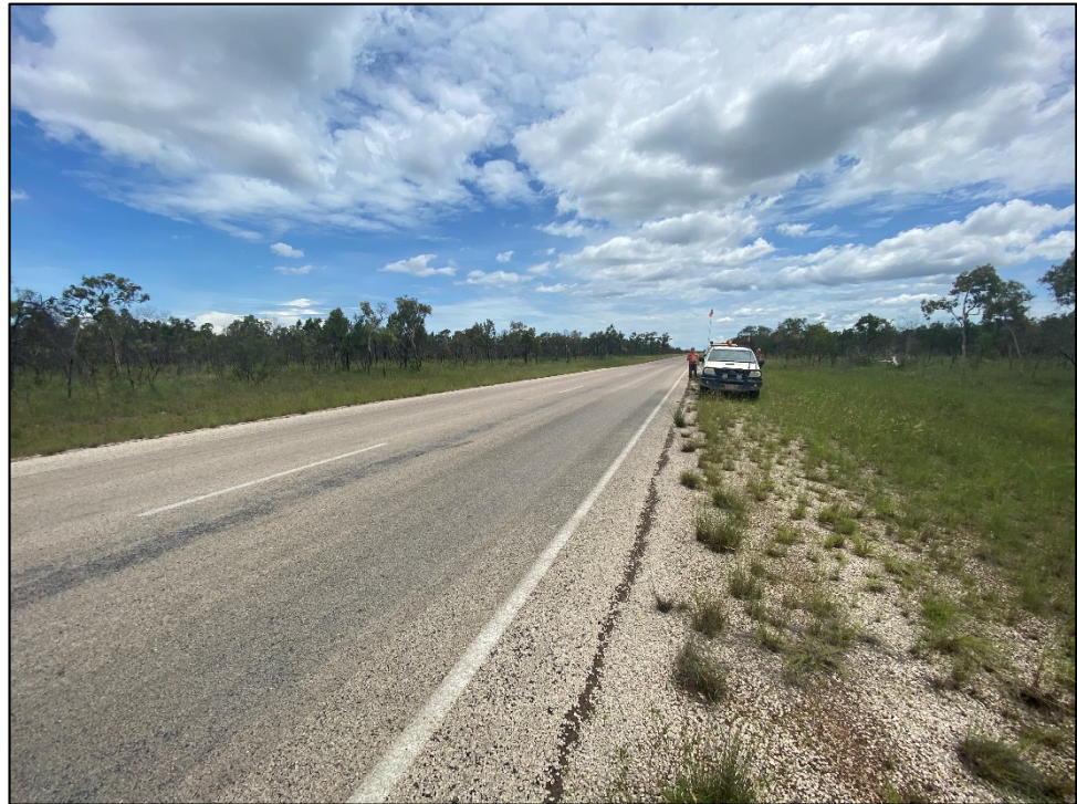
Figure 2: Concentrate observed on road prior to clean up efforts.
