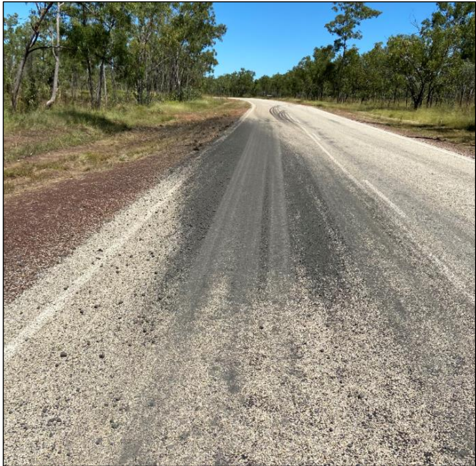
Figure 2: Bulk concentrate observed on the road surface prior to clean-up efforts.
