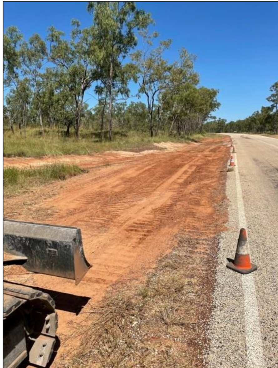
Figure 3: Incident location during clean-up efforts.
