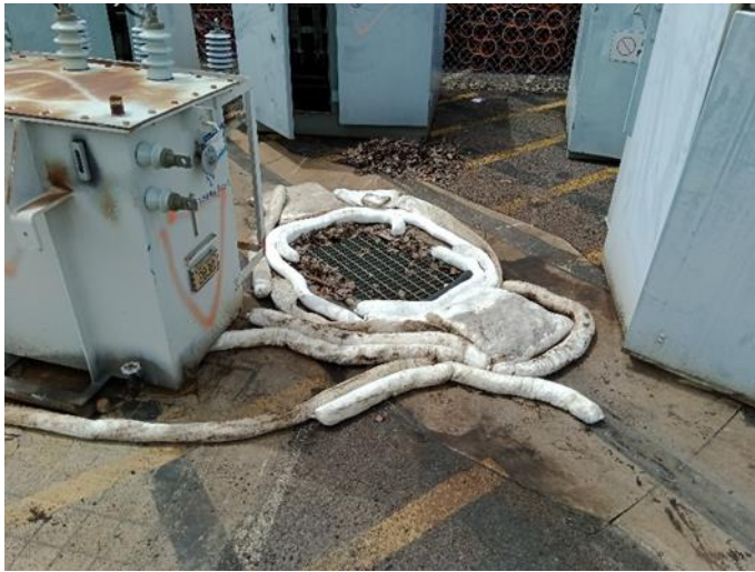
Appendix E – Photographs of the oil-filled cable spill response, deteriorated rope and area post clean-up.
