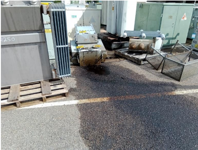
Appendix C – Photographs of the Lucy RMU spill, failed wooden pallet, spill pre and post clean-up.
