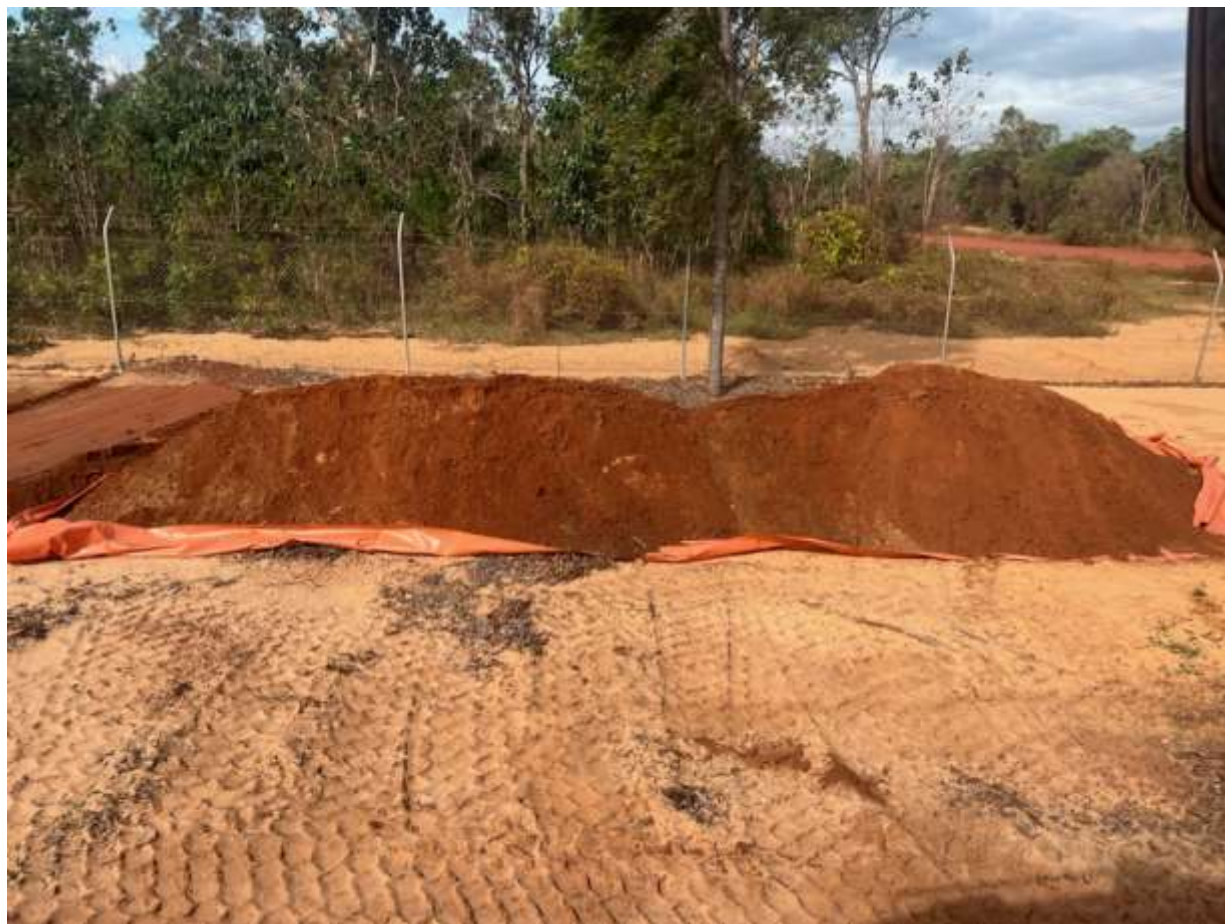
Pic 5: Immediate storage on plastic sheeting during clean-up works.
