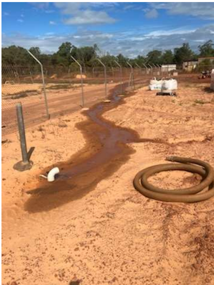
Pic 1: Fuel bund stormwater outlet
