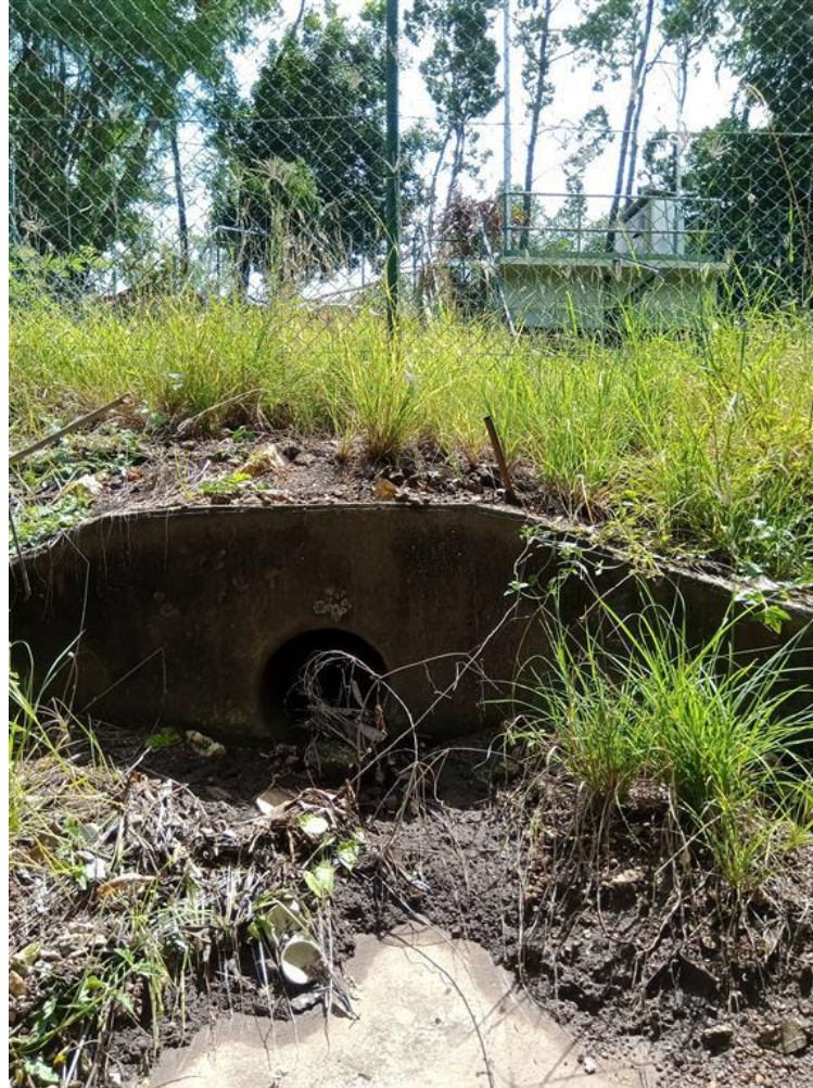
Figure 2. Photo of the stormwater and emergency overflow point headwall, with the sewage pumping station in the background.
