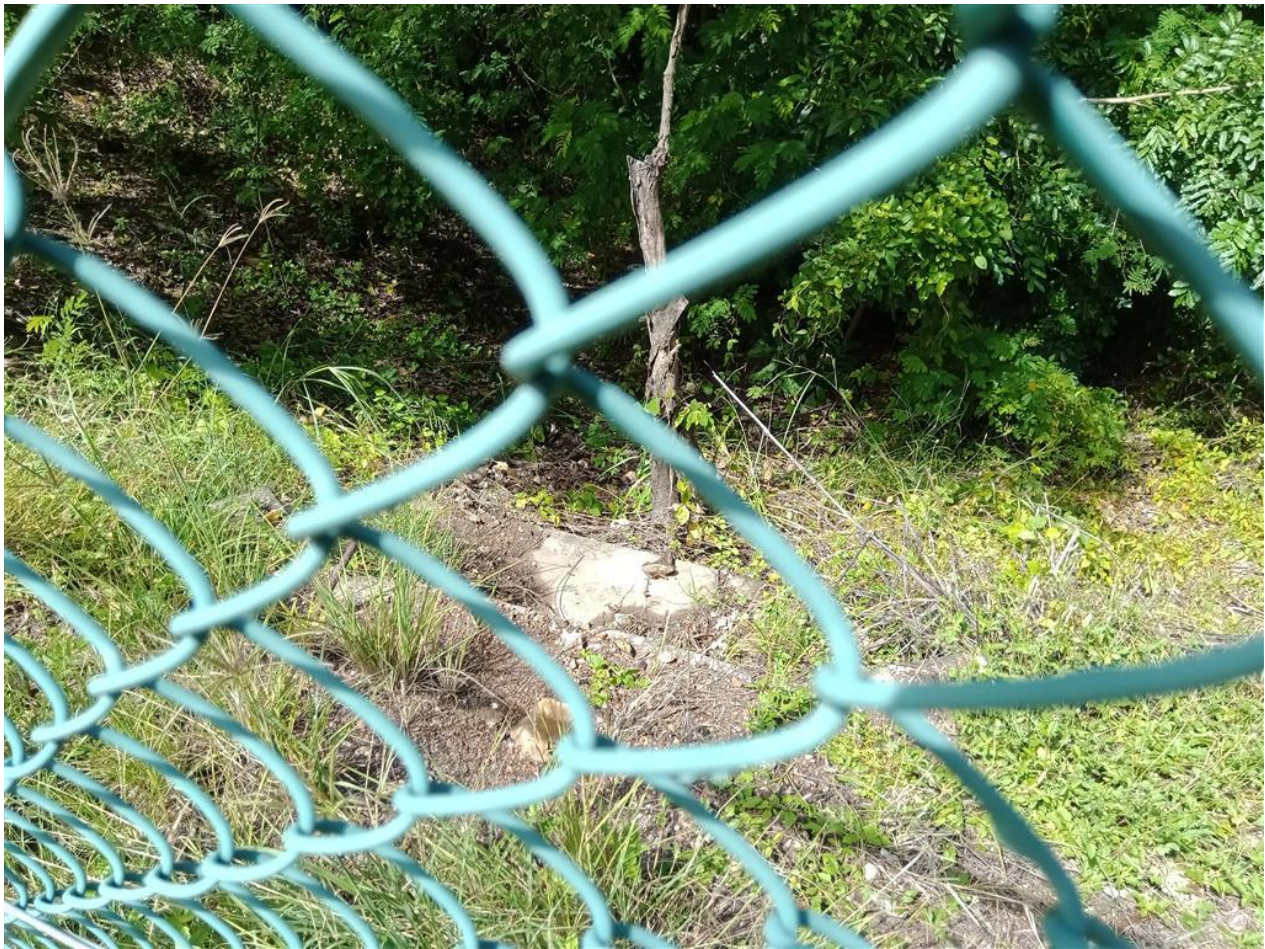
Figure 1. Photo of the stormwater drain headwall, looking from within the compound, which is also the emergency overflow point.
