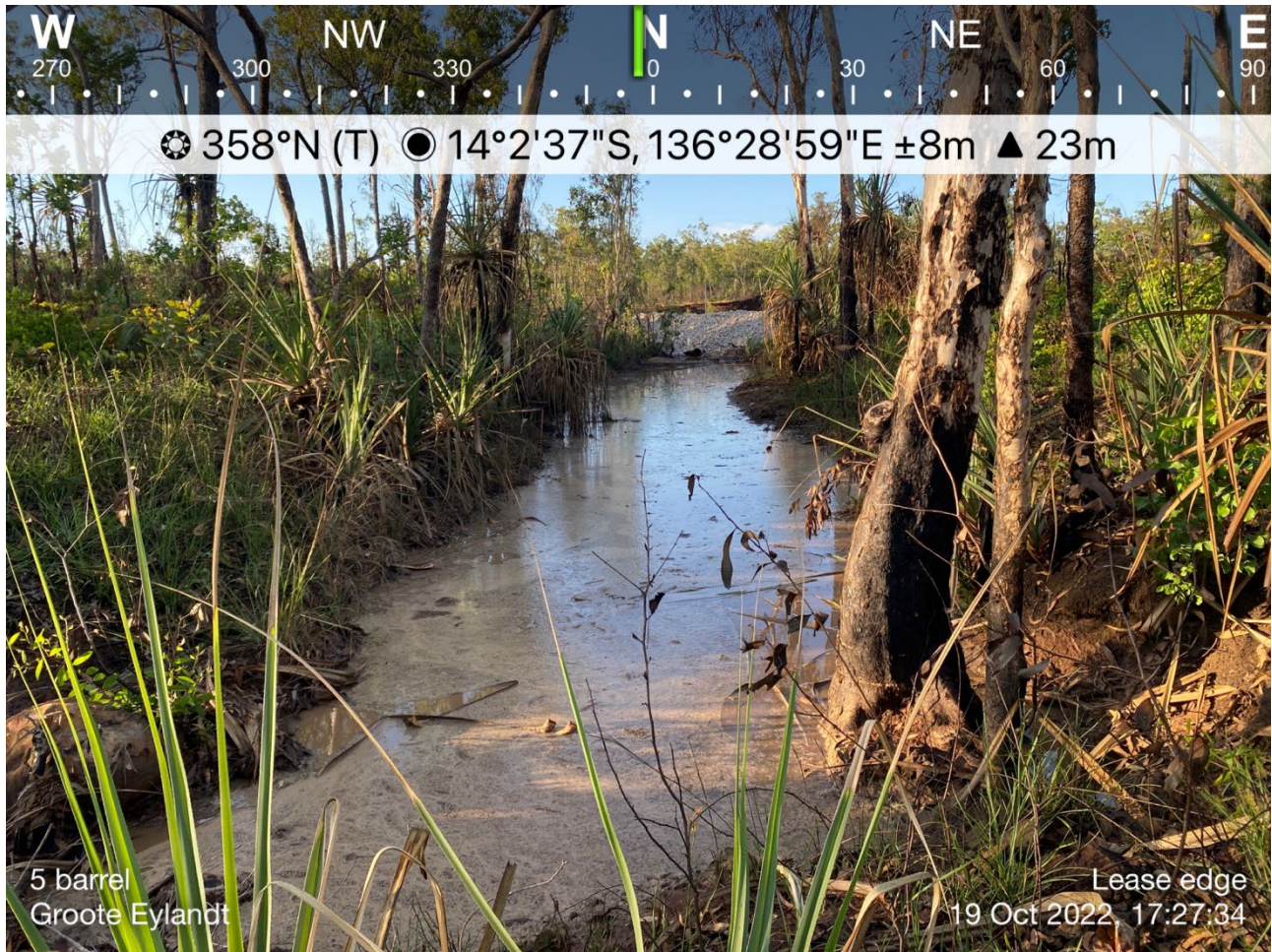
Figure 2: Sediment event in Emerald River Tributary 19 October 2022. Photograph taken from the approximate location of the lease boundary facing towards the construction area. The white rock visible in the tributary is a temporary crossing/culvert.
