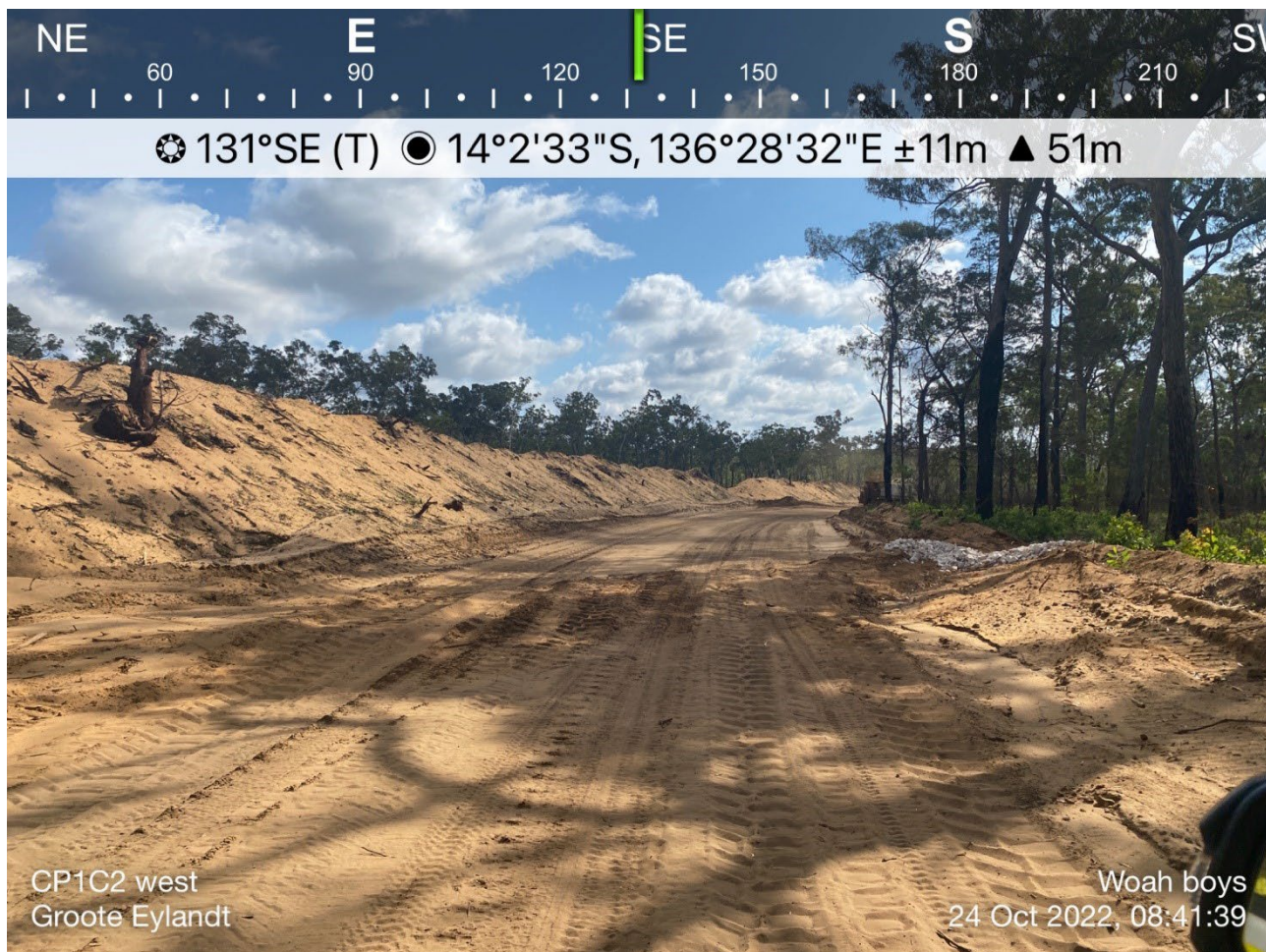
Figure 7. Improved temporary ESC: Woah boys installed to support stabilised outlets from construction access track.
