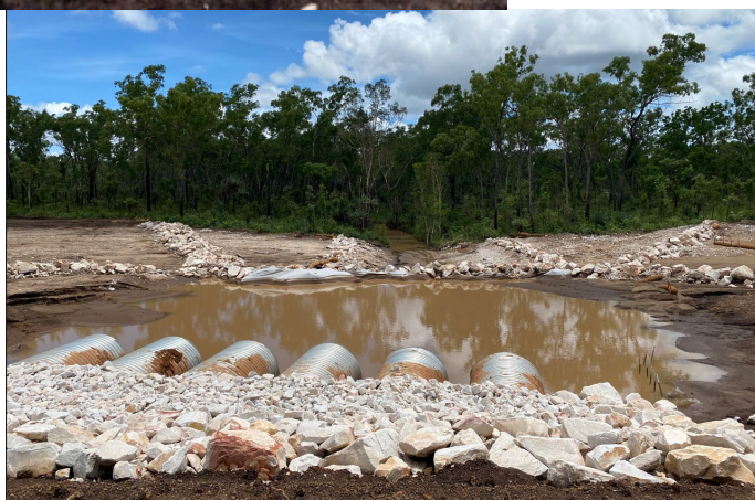
Figure 4B: 6 Barrell Culvert (CP1C2)
