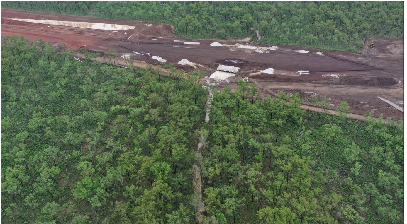
Figure 3: Sediment event in Emerald River Tributary. 14 November 2022. Photograph taken facing north (upstream) across the access authority.
