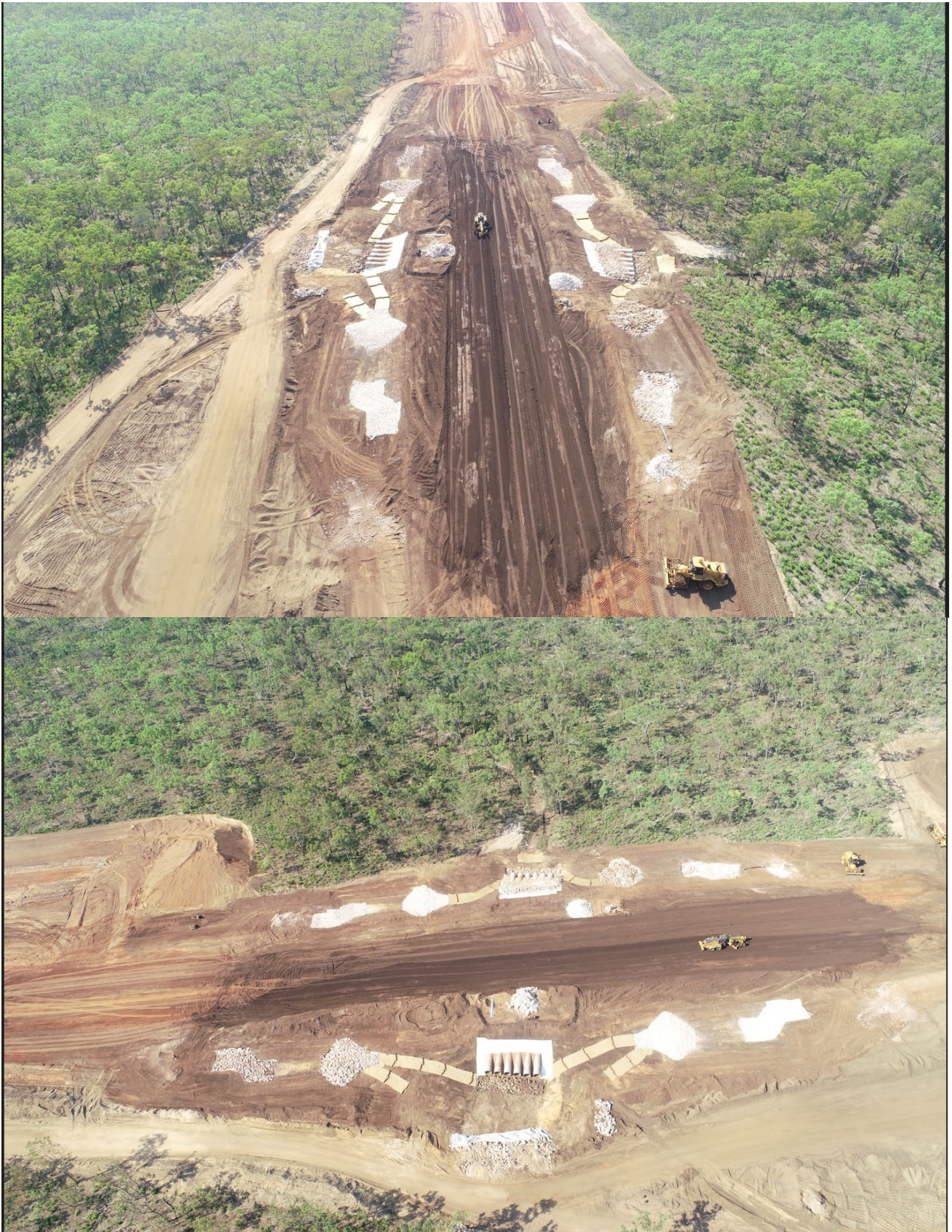
Figure 5: Sediment controls in place at the Emerald River tributary prior to the sedimentation events.
