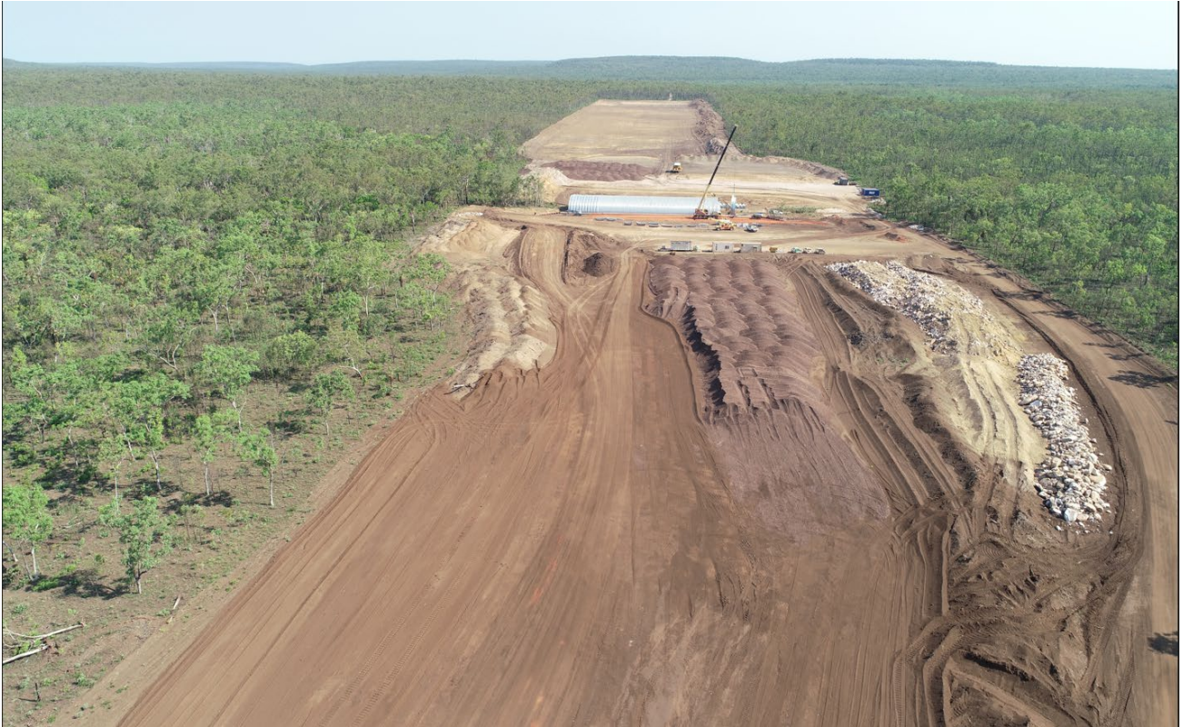
Figure 4C: Sediment controls in place at the Emerald River main channel prior to the sedimentation events.
