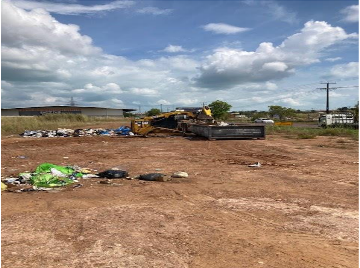
Figure 6: Load was tipped on the ground and collected with front loader into bulk bin
