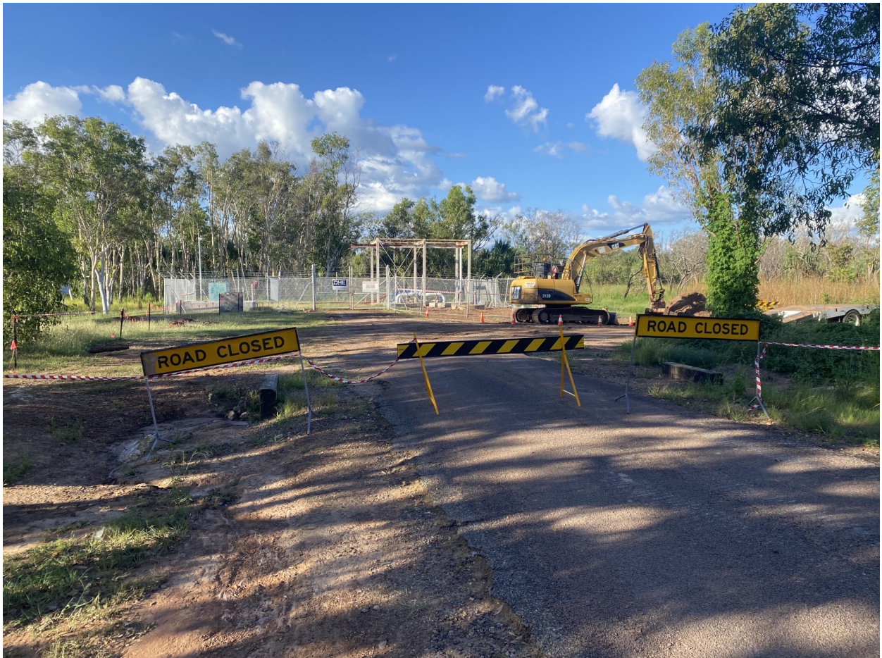
Figure 4: Site Secured with temporary Fencing
