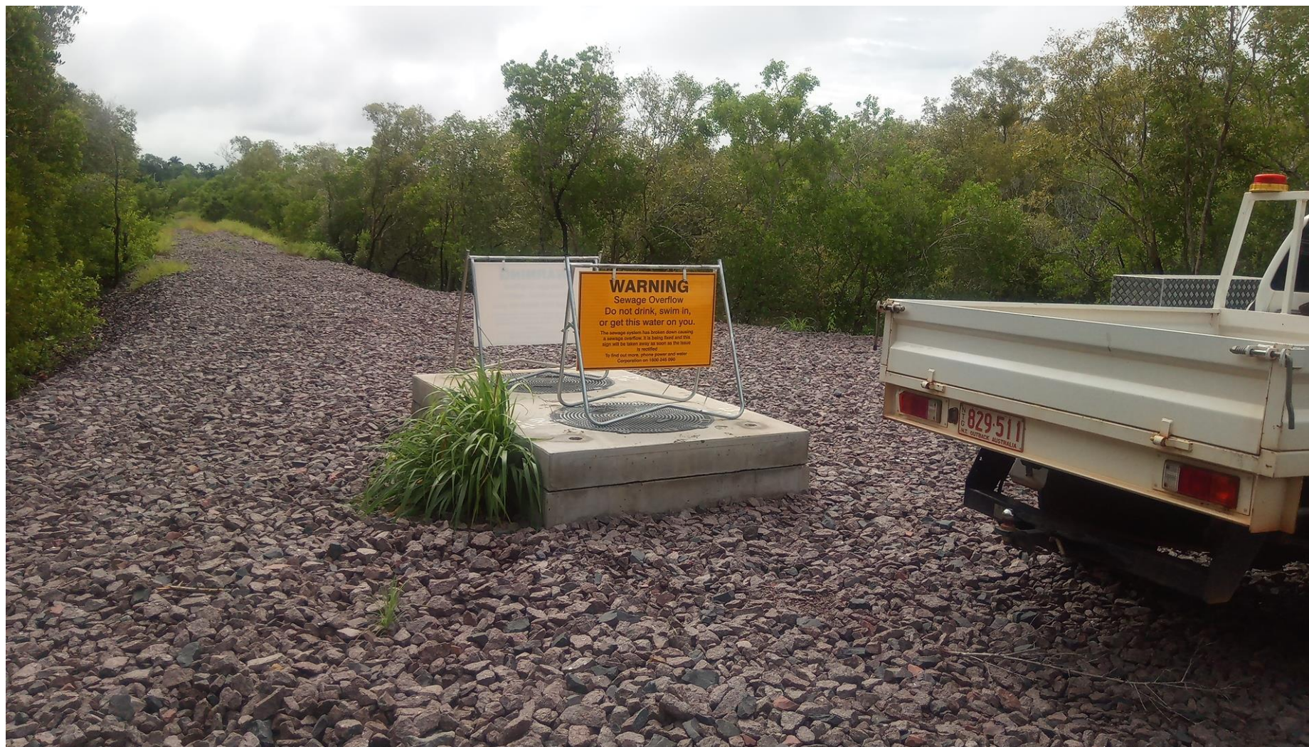
Lakeside Drive and Rapid Creek SPS Discharge Point Historical Photo dated 15/2/2021.
