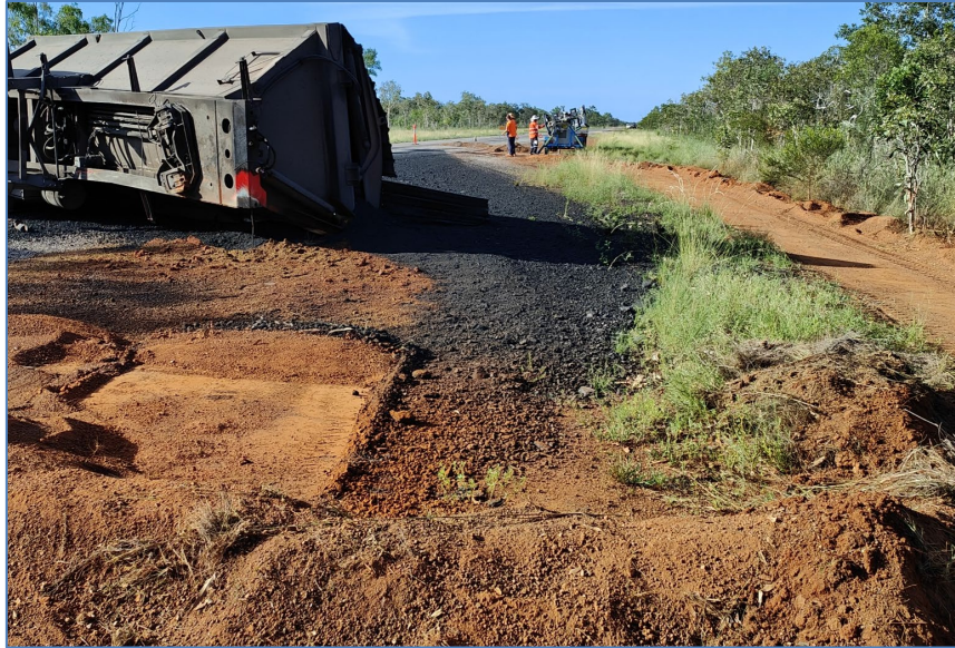
Figure 3: The bunded system around the concentrate spill area.
