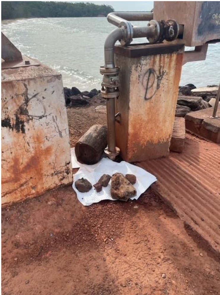
Figures 1 & 2. Milikapiti (Snake Bay) barge landing diesel fuel fill point, where the spill has come to the surface
