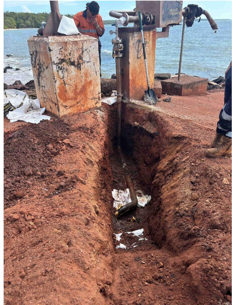
Figures 3 & 4., Where the spill has come to the surface and the excavation to expose the pipe.
