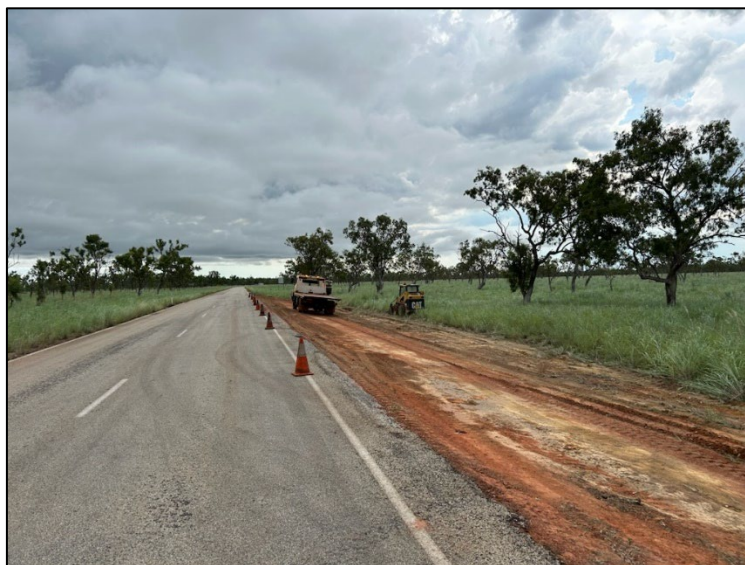
Figure 6: Grading of potentially contaminated material from the roadside.
