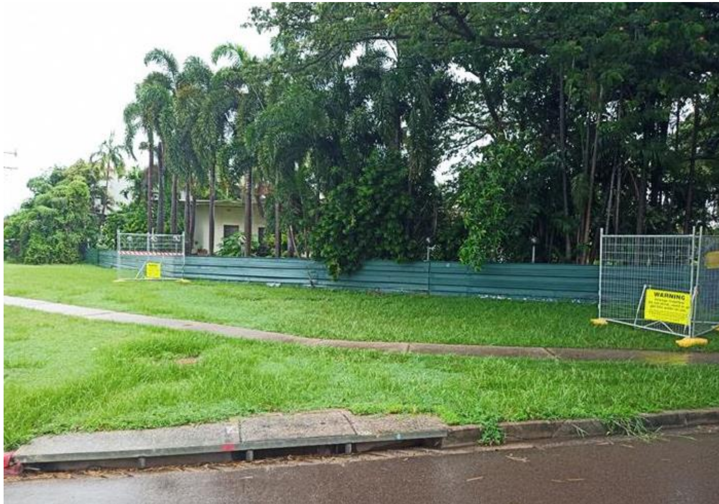
Indicative photo of the fenced access chambers on the corner of Gregory Street and East Point Road. Historical photo from 2021.
