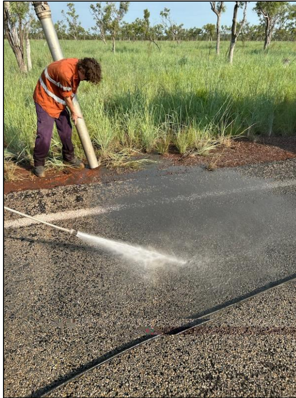
Figure 5: Removal of concentrate by a pressure hose and a vacuum truck.
