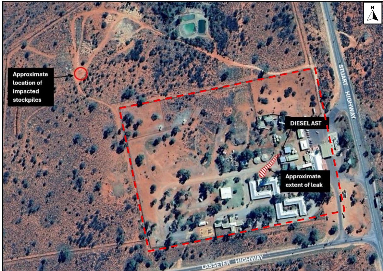
Figure 2: Diesel spill and stockpile location
