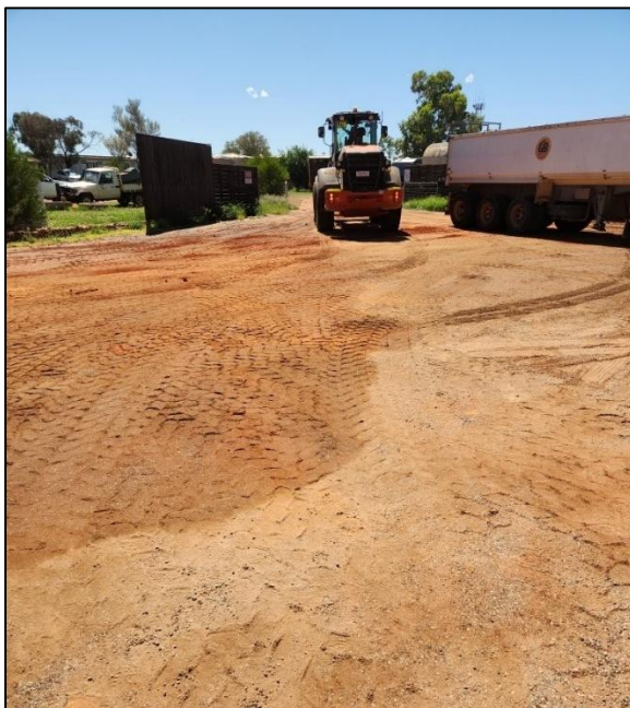
Photograph 1: View northeast across spill area during remediation works
