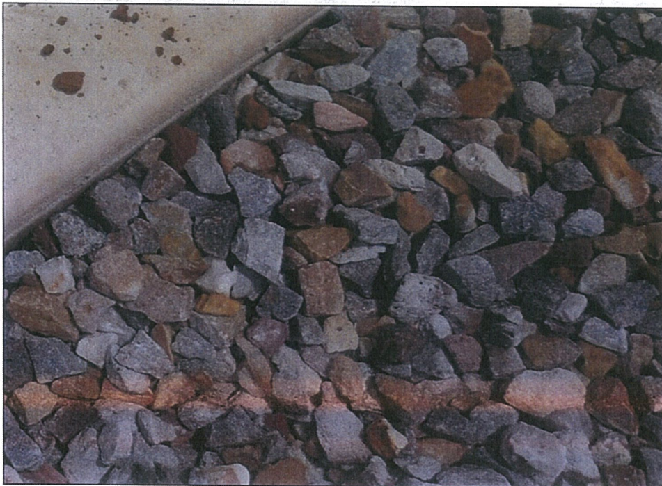
Photograph 1 – Close up of capping gravels.
