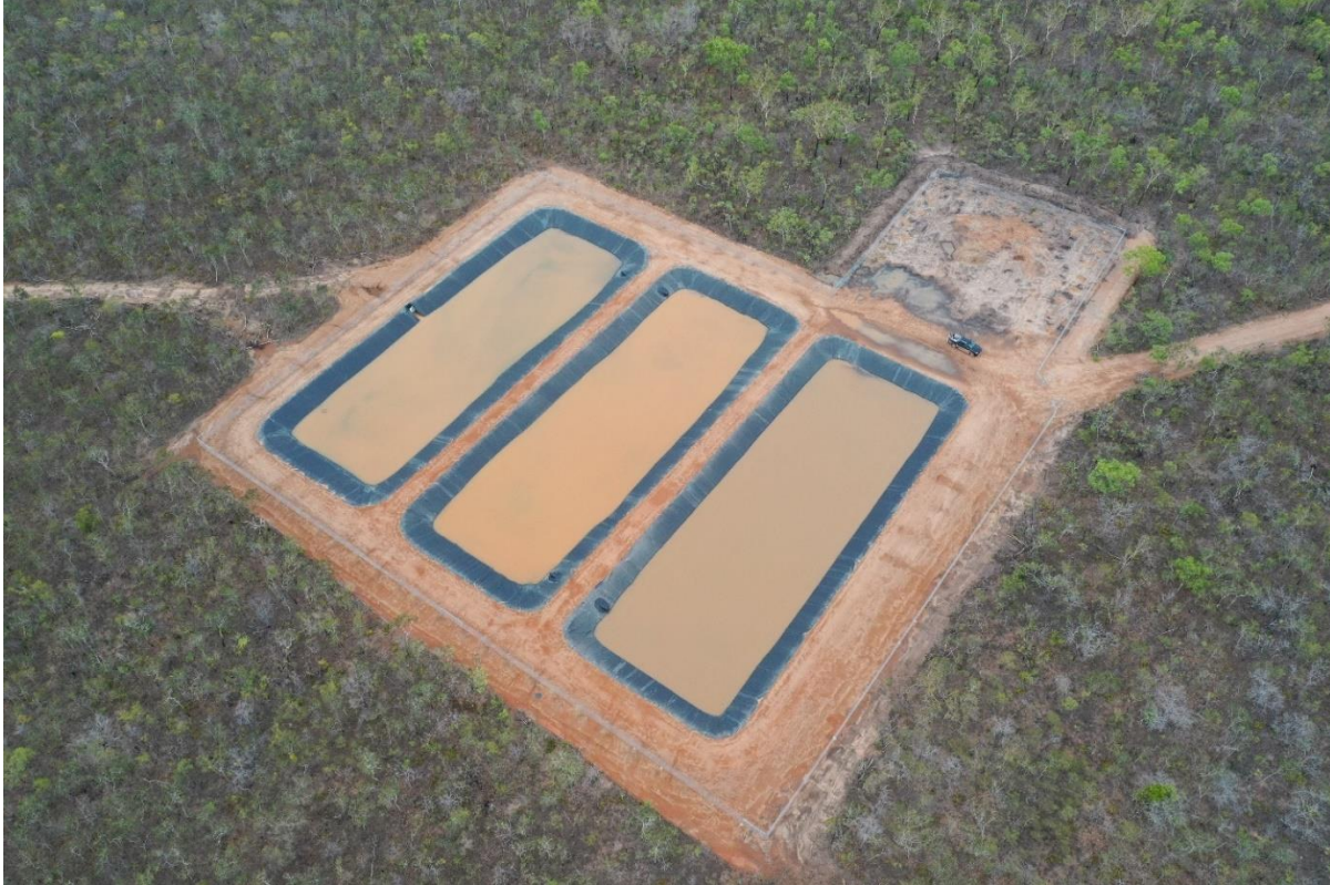
Figure 1: Discharge Settlement Ponds and Sediment Drying Area
