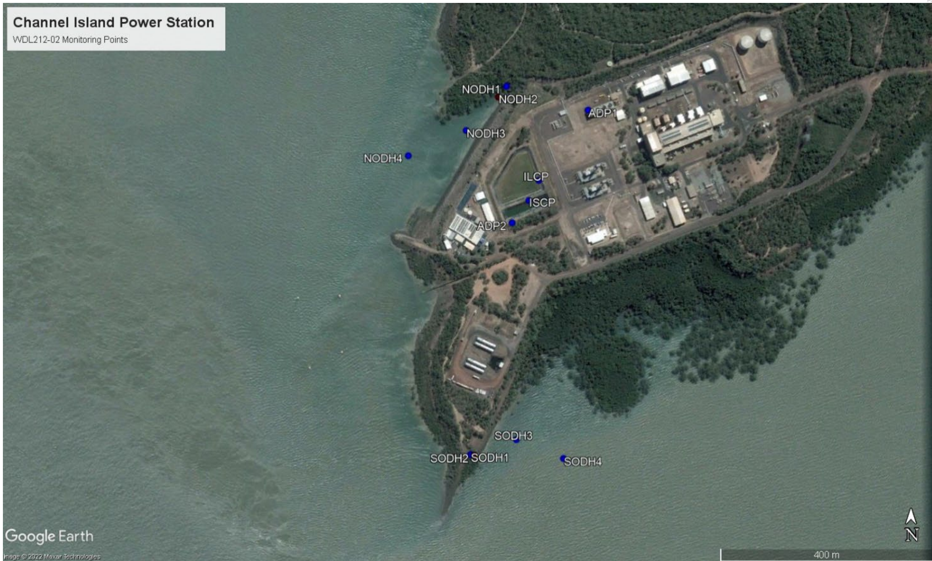
Figure 1: Aerial view of Channel Island Power Station showing WDL212-02 monitoring points.
