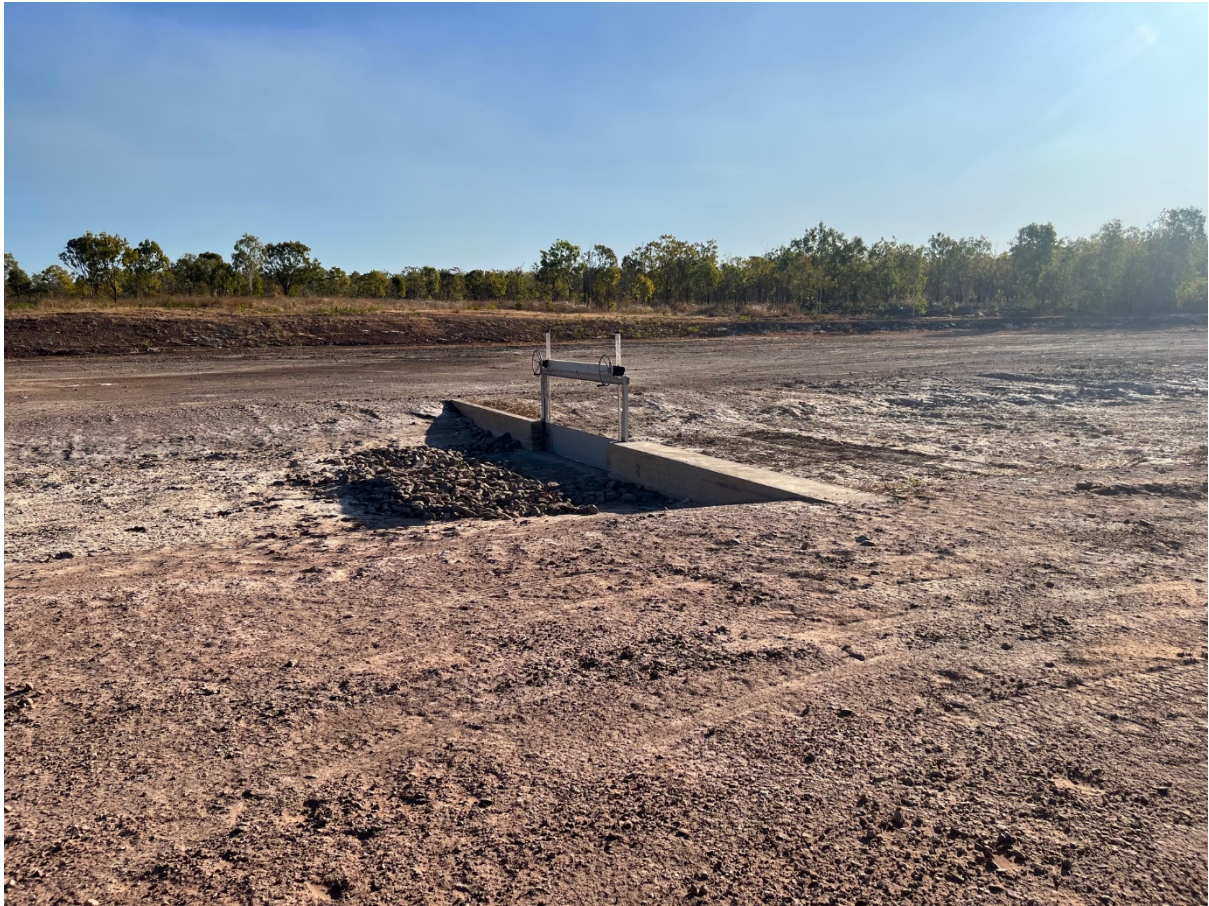
Figure 5 Installation of Weir Concrete Footing (Rock Armory)
