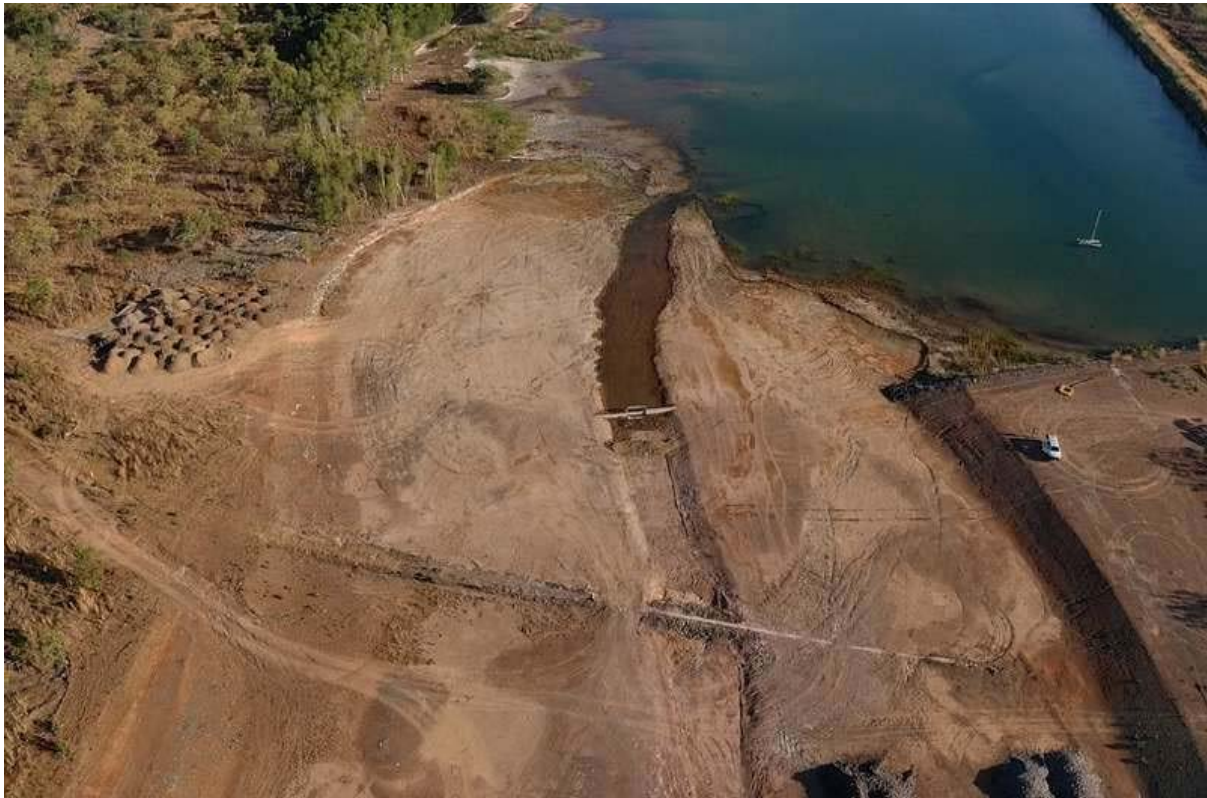
Figure 3 PCPWD Spillway Post Clean up
