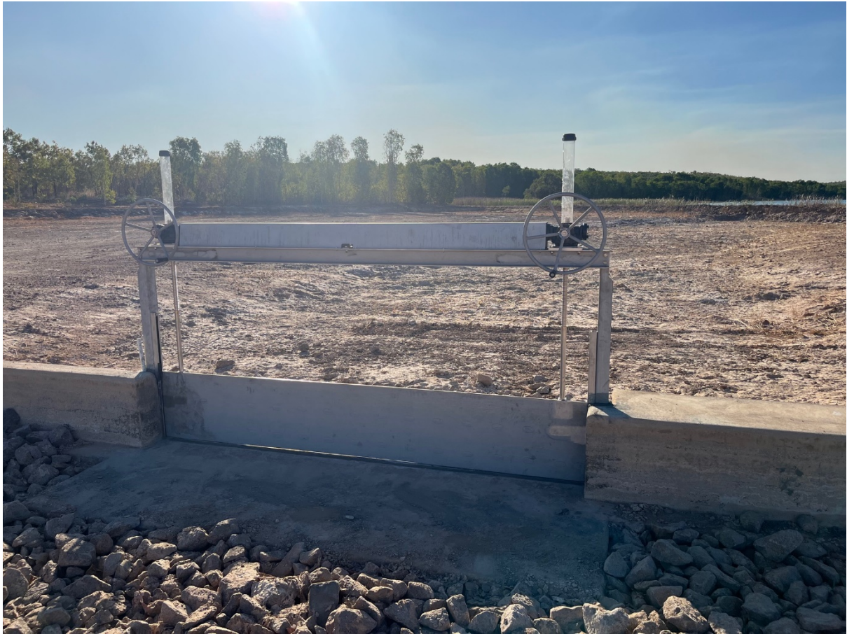
Figure 4 Installation of Sluice Gate
