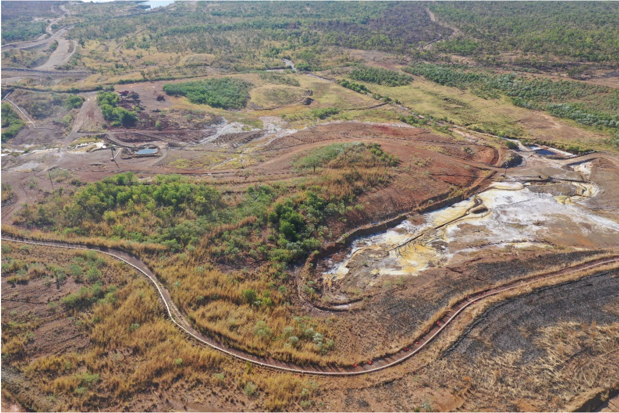
FIGURE 1 MINE WATER DAM ROCK DRAIN INSTALLATION
