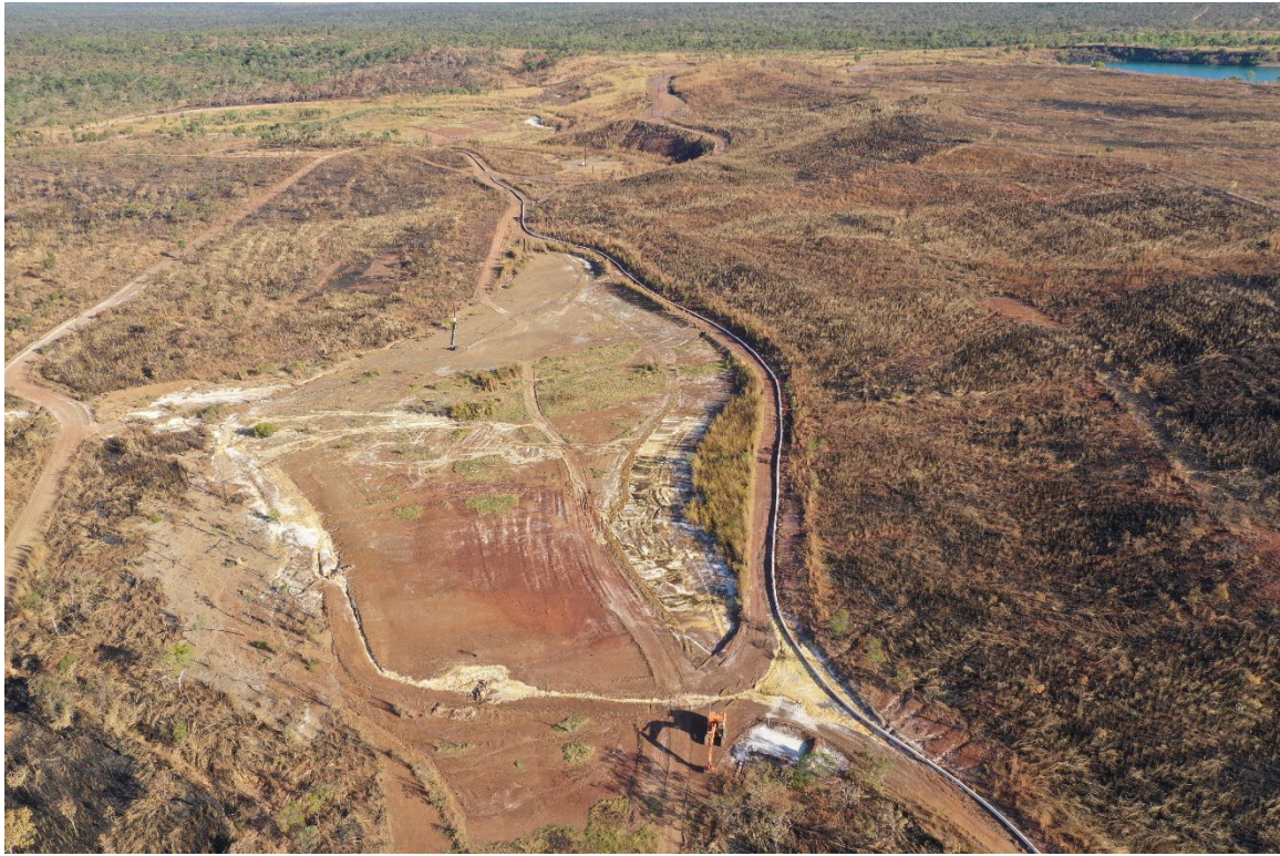
FIGURE 2 ACID POND 4 COMPLETED ROCK DRAIN INSTALLATION
