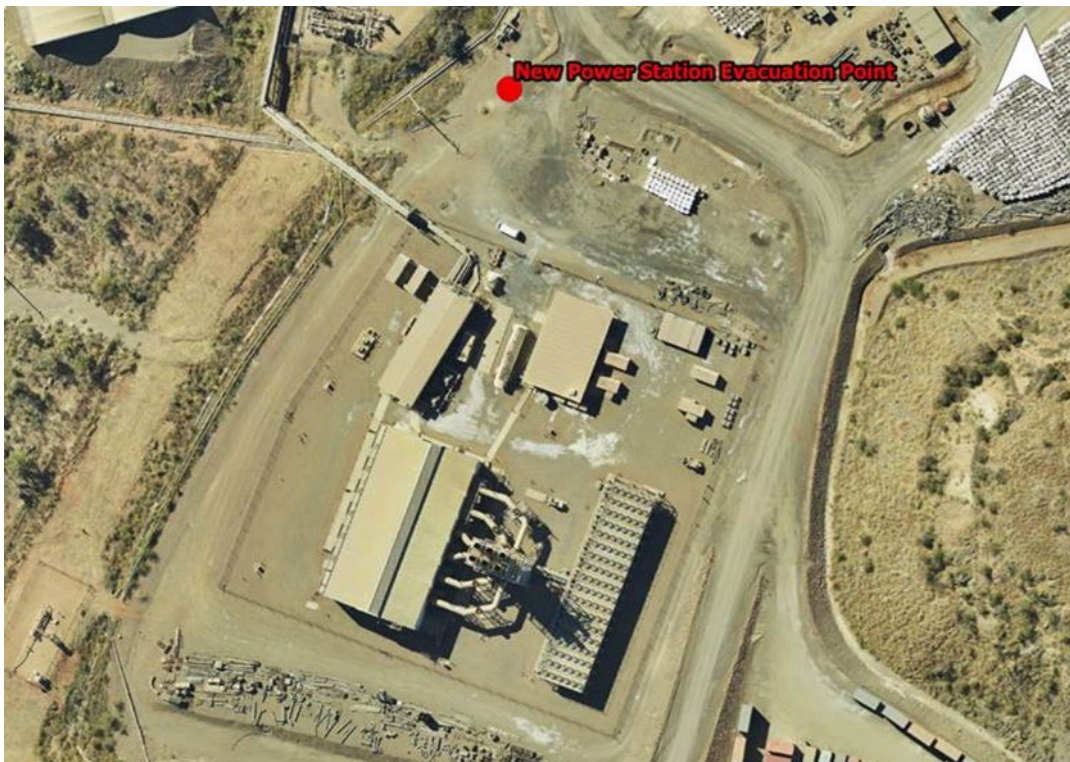
Figure 11 - Evacuation Point New Power Station
