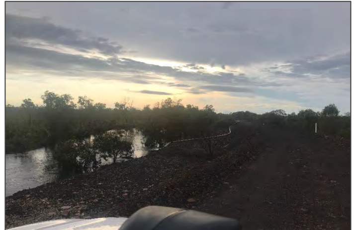
Image 2: View of unauthorised discharge point 2. 16/2/21 7:10 am.
