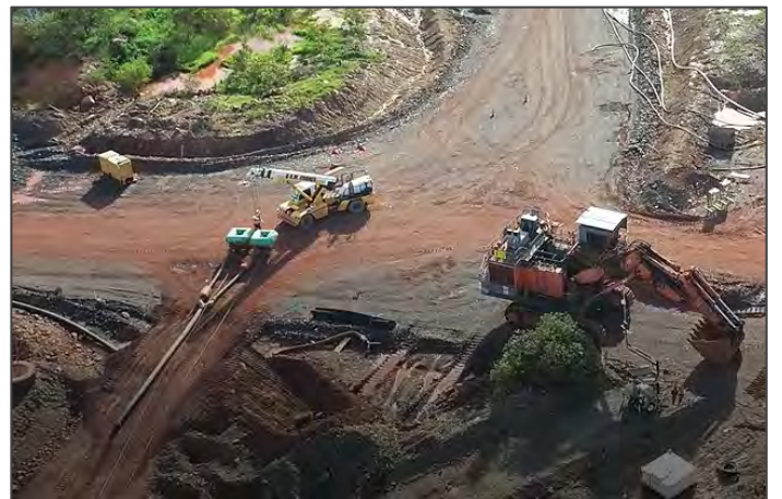
Image 4: Relocation of 2 x 90KW pumps from FE1 to FE2 14/2/21 ~5:20 pm.
