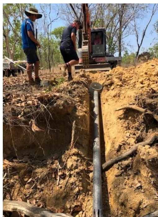
RRSW24 telemetry station construction installing steel housing to creek (Nov 2021) Rustlers Roost
