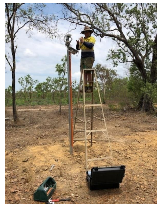
RRSW24 telemetry station construction installing satellite and solar panel (Nov 2021) Rustlers Roost
