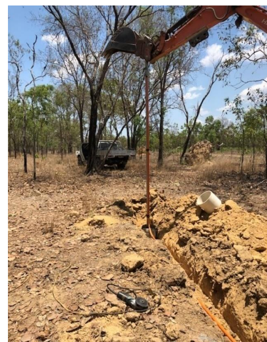
RRSW24 telemetry station construction laying conduit (Nov 2021) Rustlers Roost
