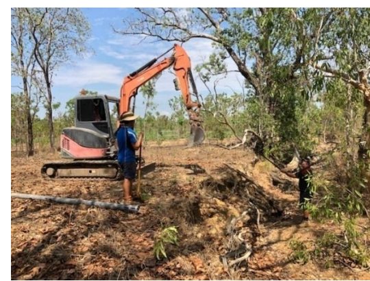
RRSW24 telemetry station construction digging conduit line (Nov 2021) Rustlers Roost
