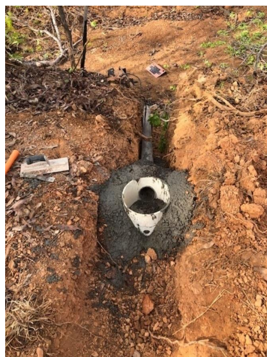
RRSW24 telemetry station construction installing access connection pit (Nov 2021) Rustlers Roost
