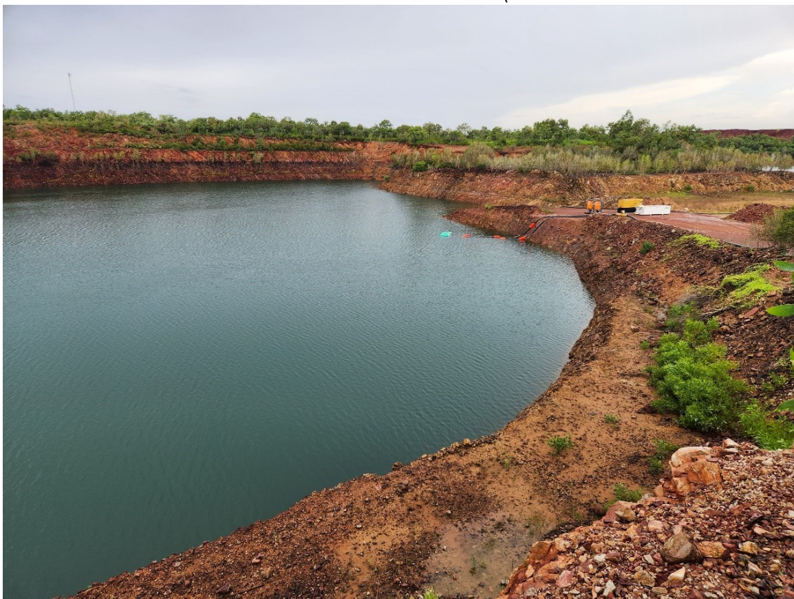
Overlooking Pump set up in Rustlers Roost Main Pit
