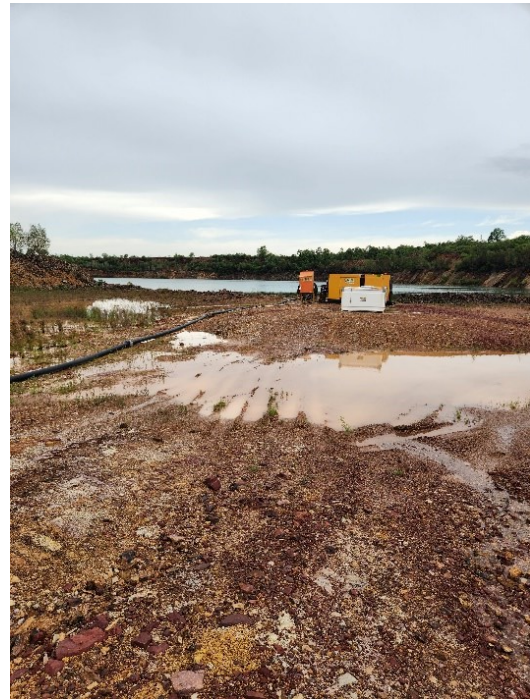
Staging water pump and generator located on wall between Backhoe Pit and Rustlers Roost Main Pit (Jan 2023)
