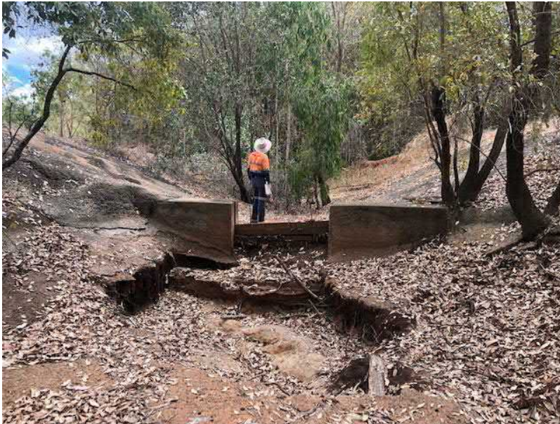
Figure 2 Oxbow Wetlands weir gate
