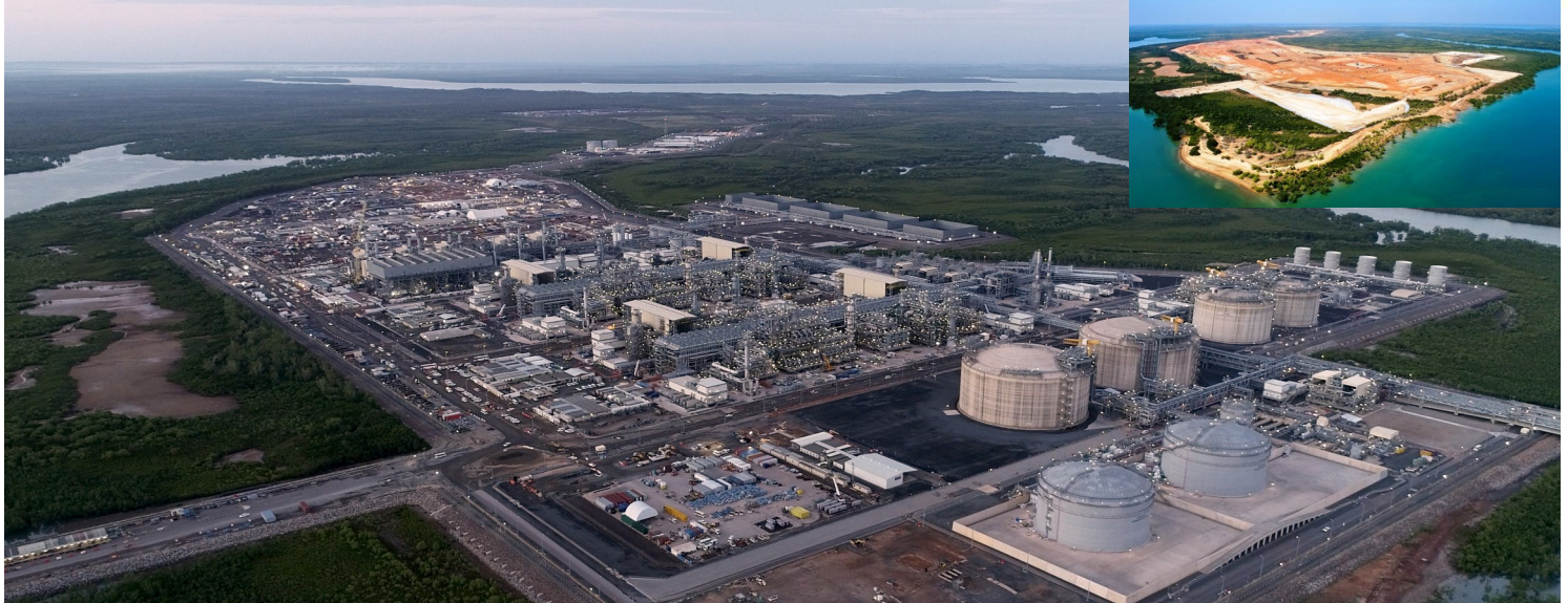
Construction of the Ichthys Project Onshore LNG Facilities is almost complete. Inset: Bladin Point in September 2012.
