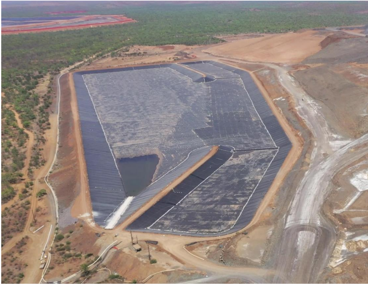
Plate 5: HDPE-Lined SPROD (Looking West)
