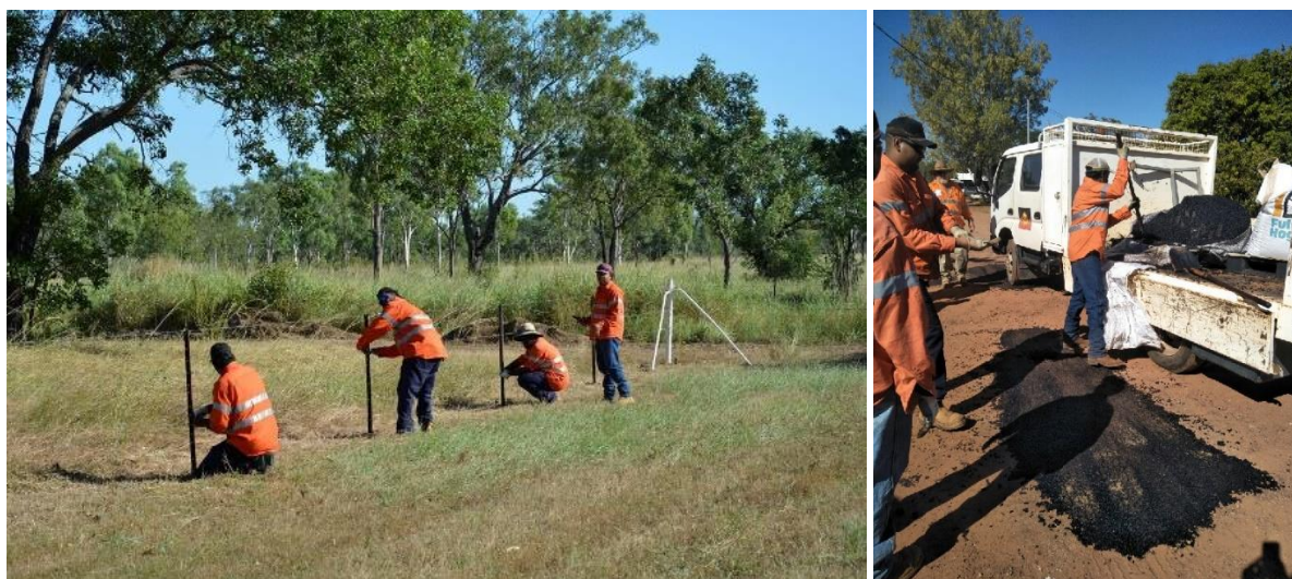
Plate ES7: Local Workforce Installing Fencing (left), and Filling Potholes (right)
