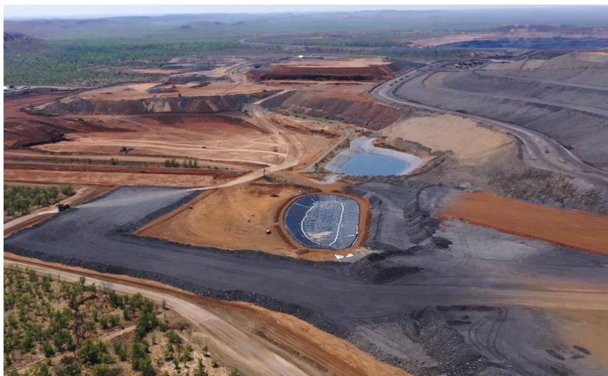
Plate 2: Central West Charlie Sump (Looking South)
