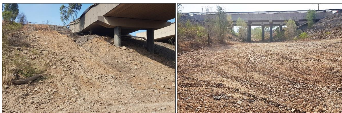
Plate ES4: Sediment Removal from Barney Creek
