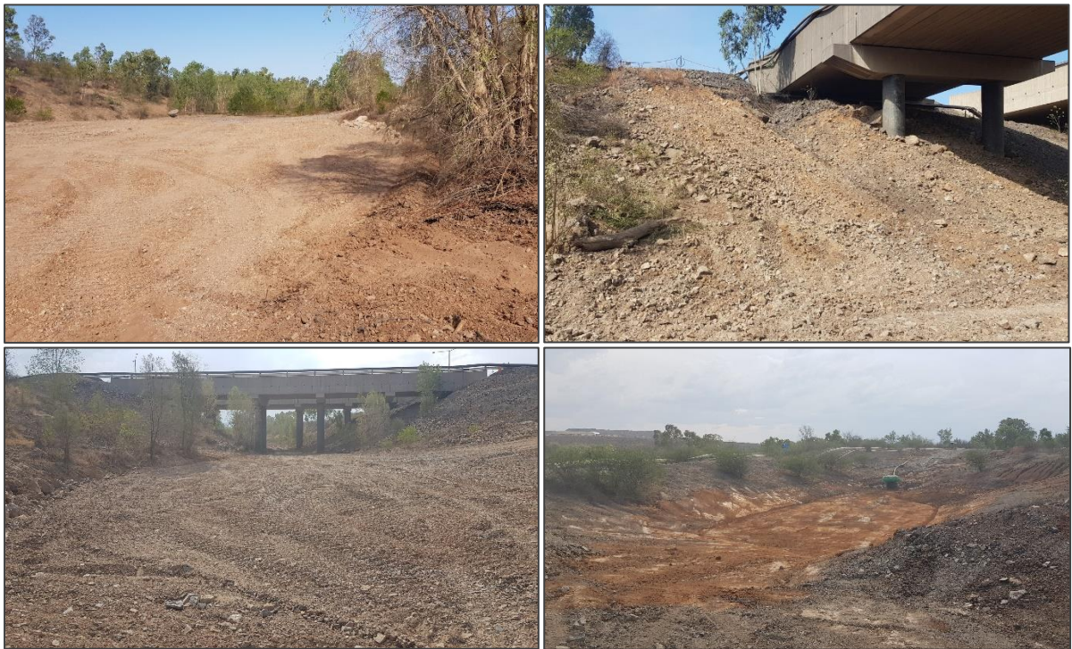
Plate 22: Sediment Removal from Barney Creek and Barney Creek Bridge Sump
