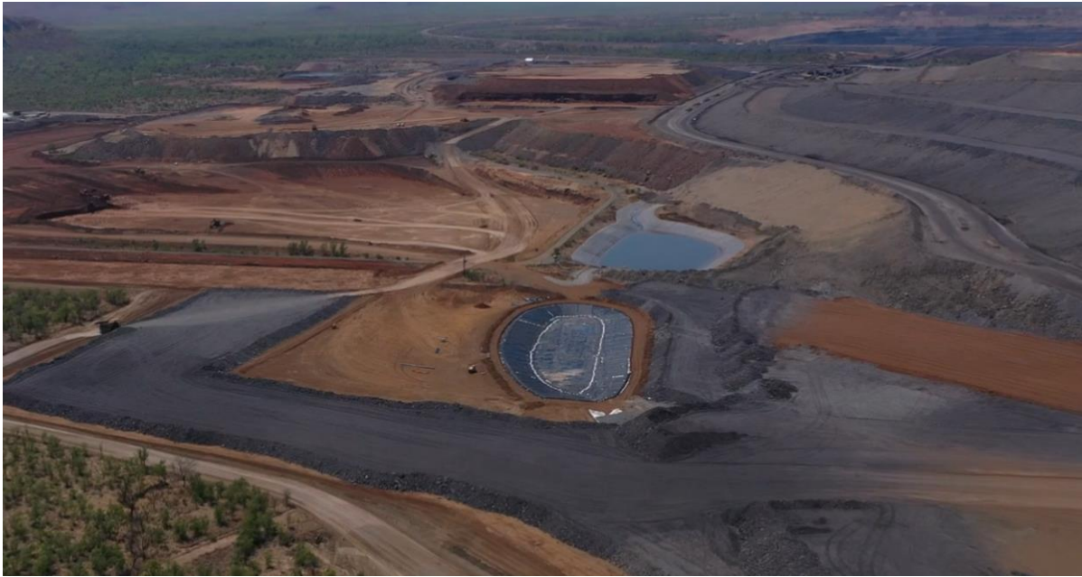
Plate ES1: Lining of Central West Charlie Sump at the North Overburden Emplacement Facility
