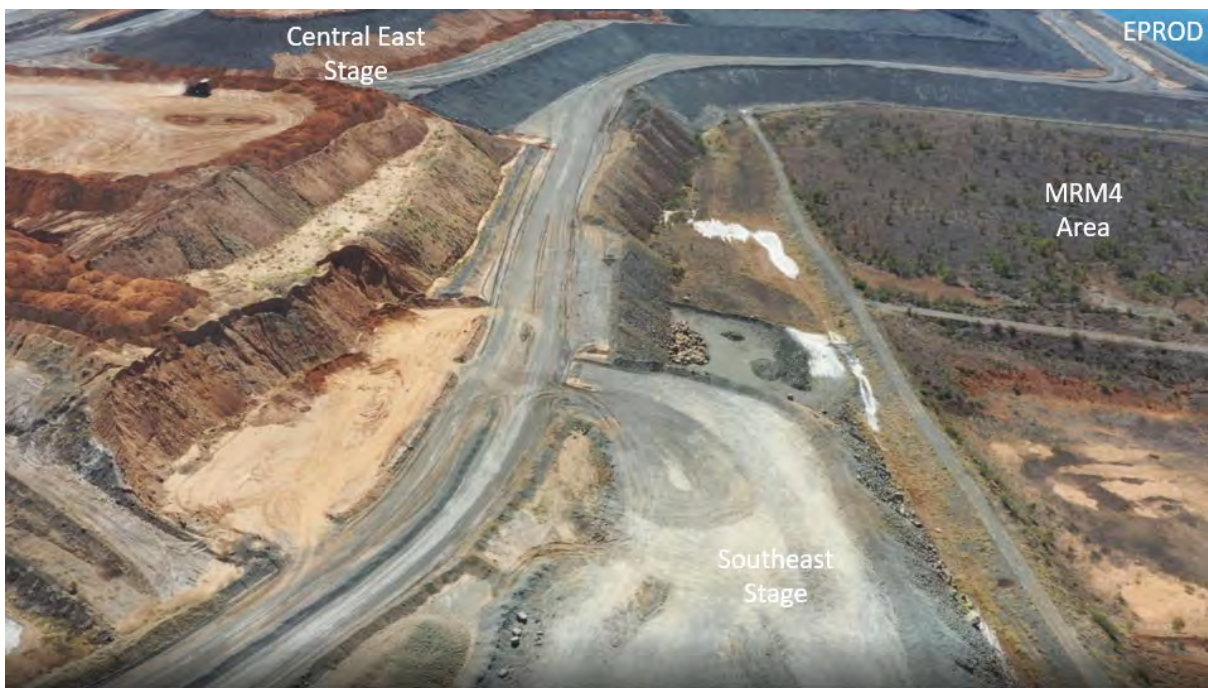
Plate 4: MRM4 Area Drone Photo – 24 July 2022
