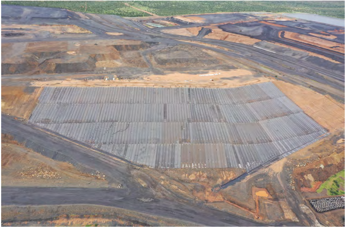
Plate 7: NOEF Rehabilitation Trial Area – Drone Shot
