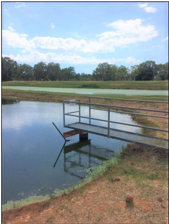
Figure 15: Barunga Pond 5, Final outfall (PWC 2021)
