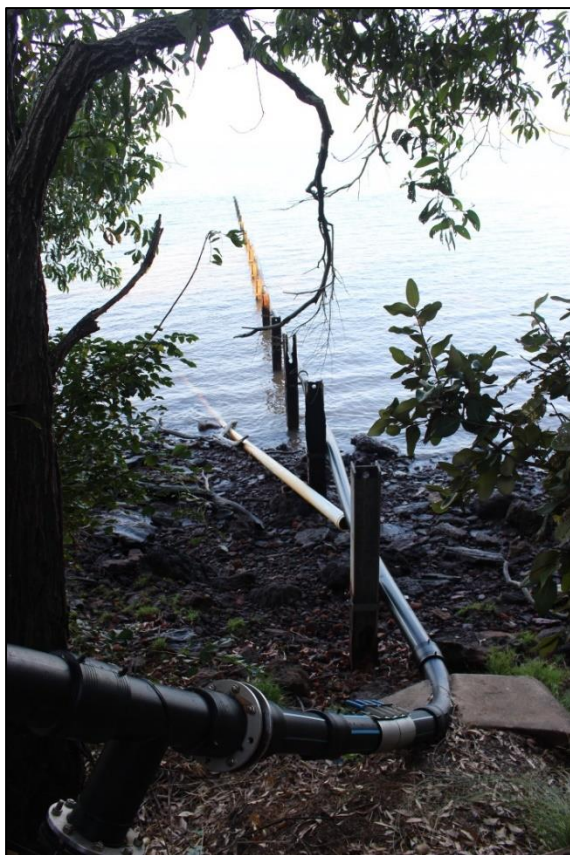
Figure 14: Milikapiti outfall pipe during ERA inspection (PWC 2017)
