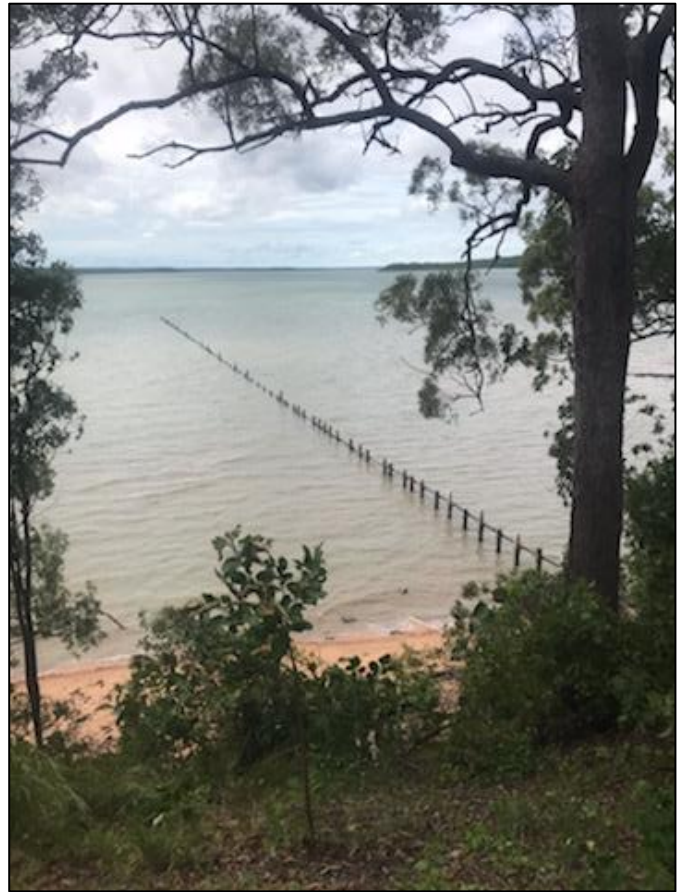
Figure 8. Milikapiti discharge point outfall (PWC 2021)
