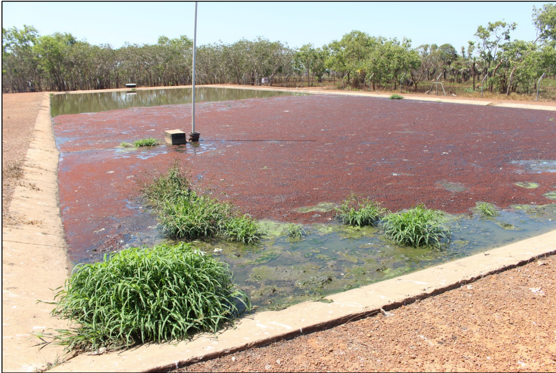
Figure 13. Nganmarriyanga WwTP Pond 1 (PWC 2017)
