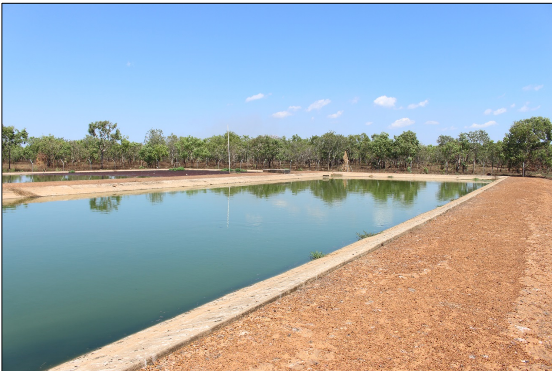
Figure 14. Nganmarriyanga WwTP Pond 2 (PWC 2017)
