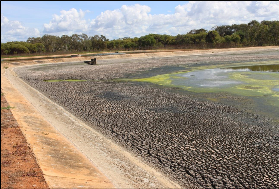
Figure 12: Pond drained to be desludged (PWC 2017)
