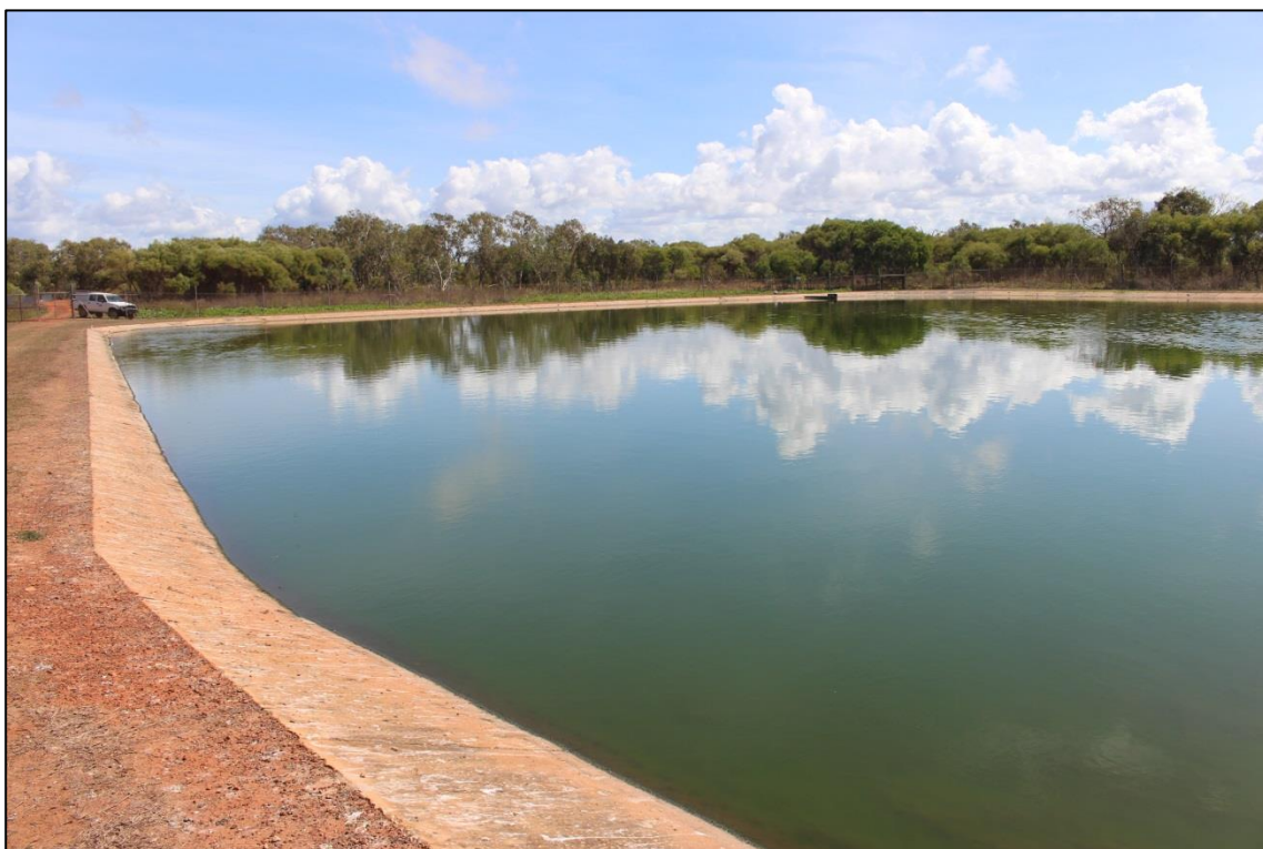
Figure 11: Numbulwar WwTP (PWC 2017)
