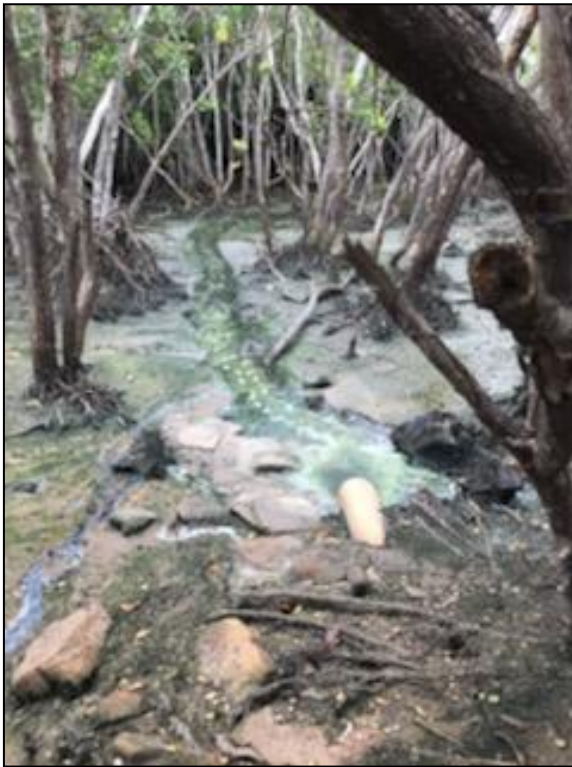
Figure 7: Final discharge point (PWC 2021)
