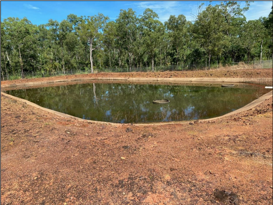
Figure 12. Pirlangimpi WwTP Pond 2 – Wet Season 2021 (PWC 2021)
