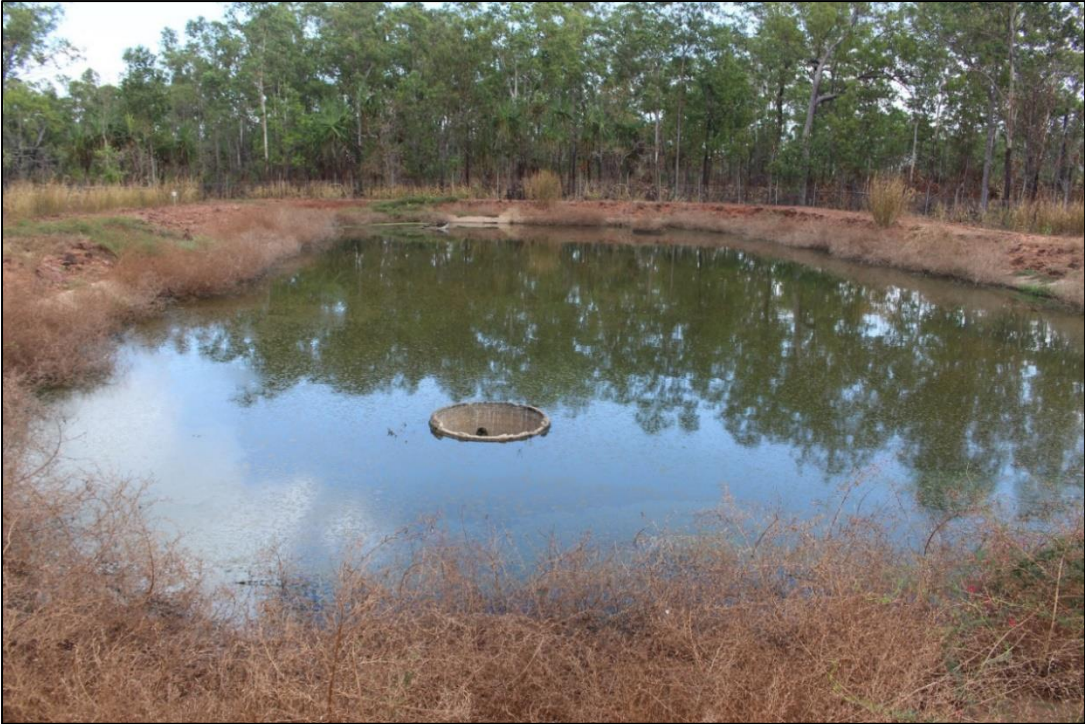
Figure 11. Pirlangimpi WwTP Pond 2 (PWC 2017)
