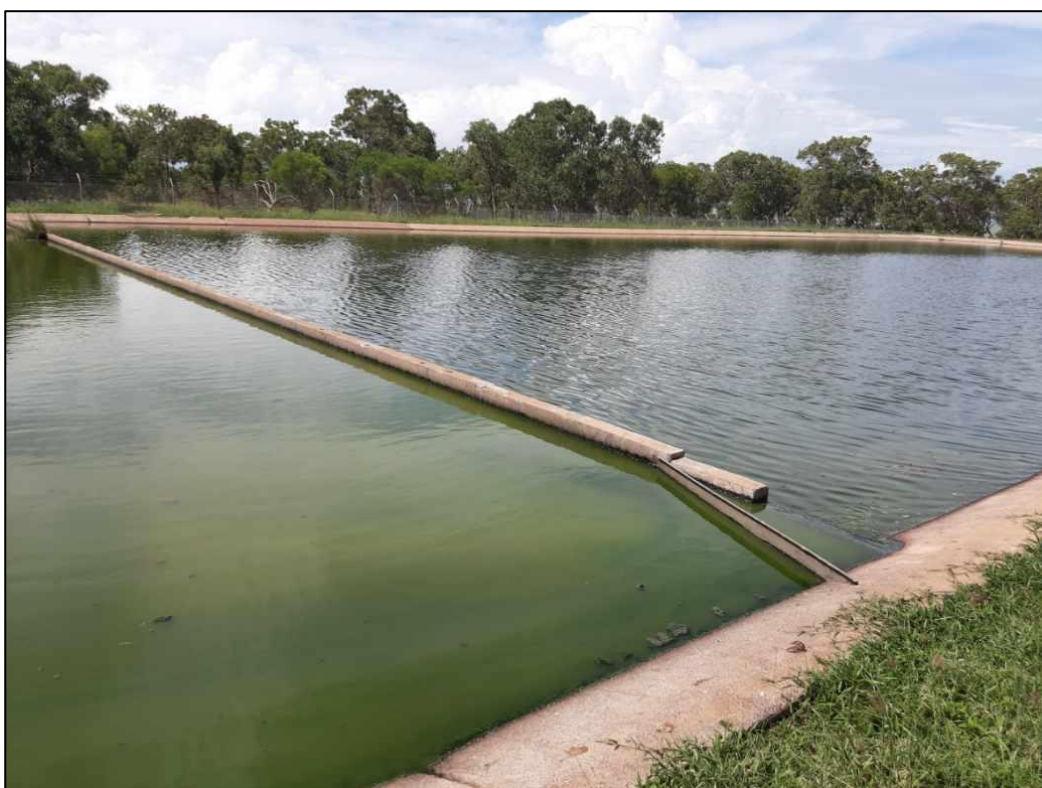
Figure 13. Warruwi WwTP Pond 1 (left) and Pond 2 (right) (PWC 2021)
