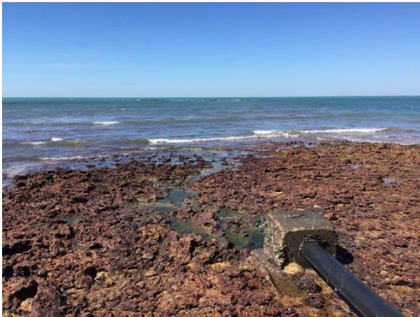
Figure 5. Warruwi WwTP ocean outfall at low tide (PWC 2016)
