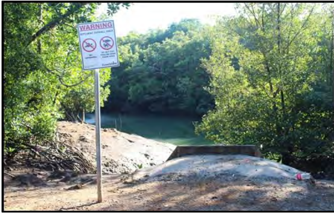
Figure 5. Wurrumiyanga WwTP discharge outlet (PWC 2017)
