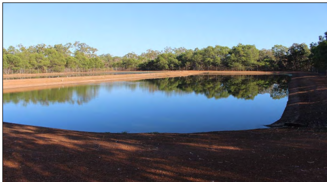
Figure 16. Wurrumiyanga WwTP Pond 2 and Pond 3 (foreground) (PWC 2017)
