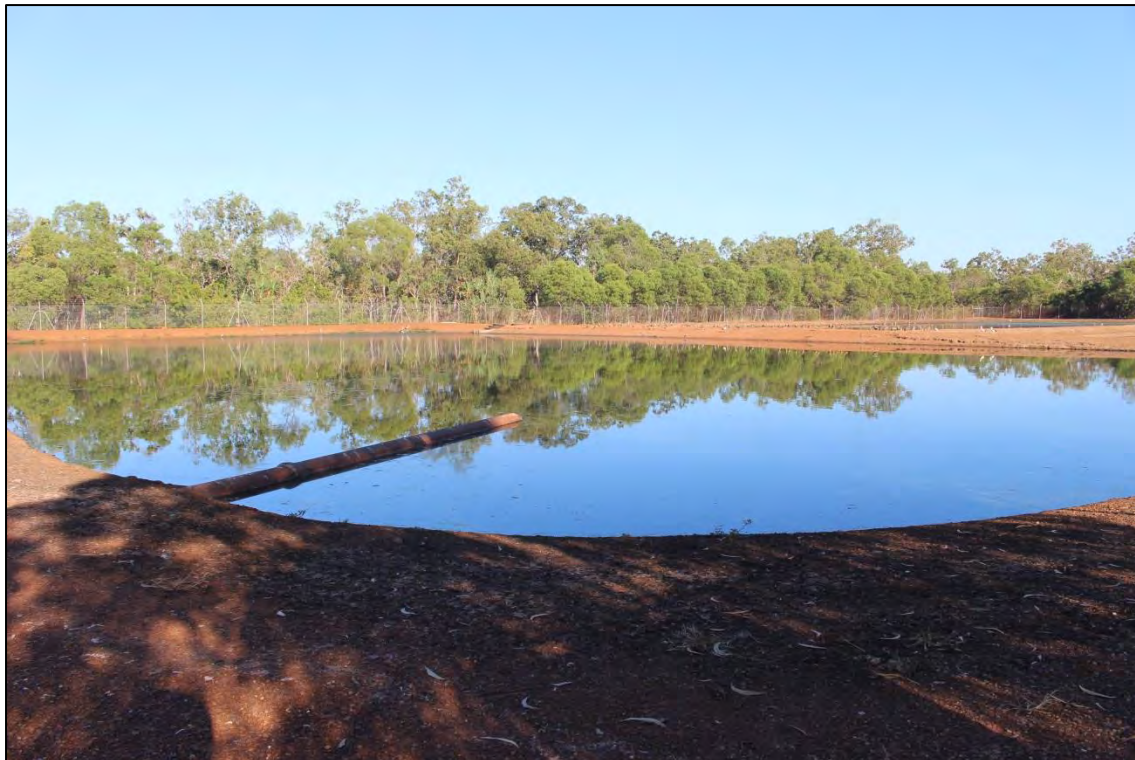
Figure 15. Wurrumiyanga WwTP Pond 1 (PWC 2017)
