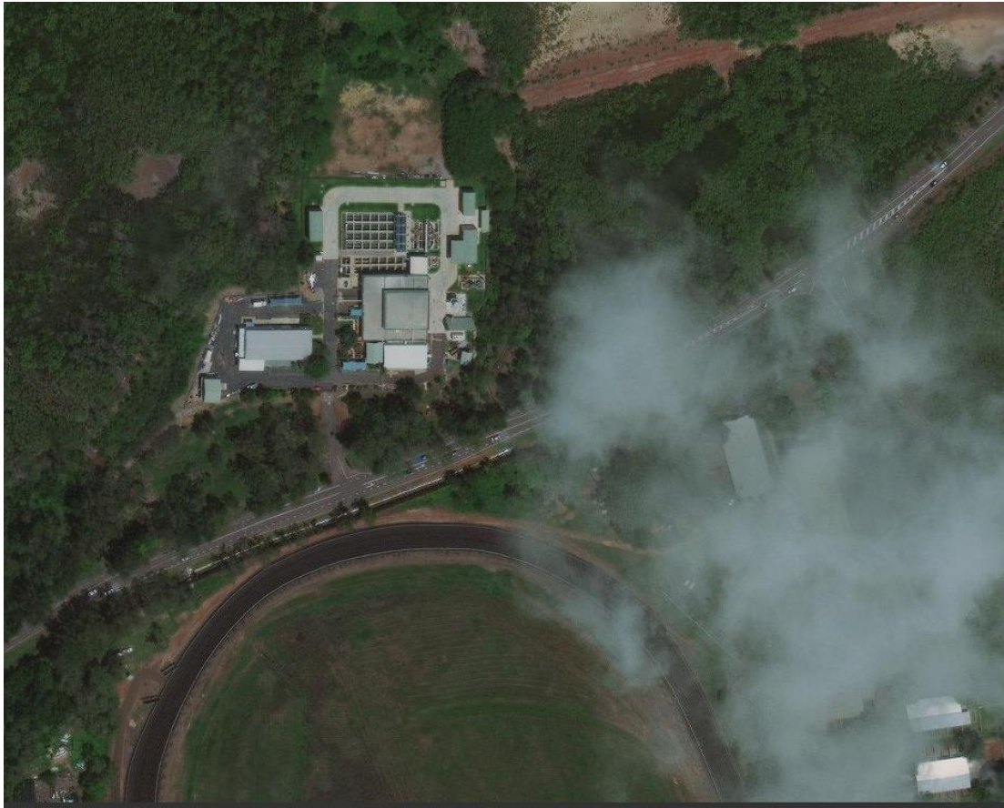
Figure 2: Ludmilla Wastewater Treatment Plant Dick Ward Drive Ludmilla
