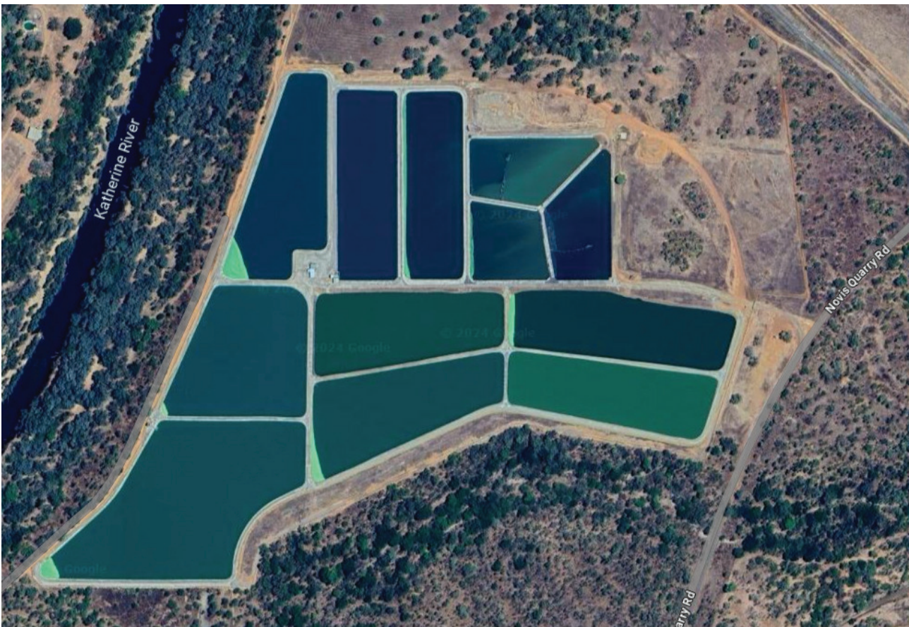
Figure 1: Katherine Waste Stabilisation Ponds (Google Image, 2022)
