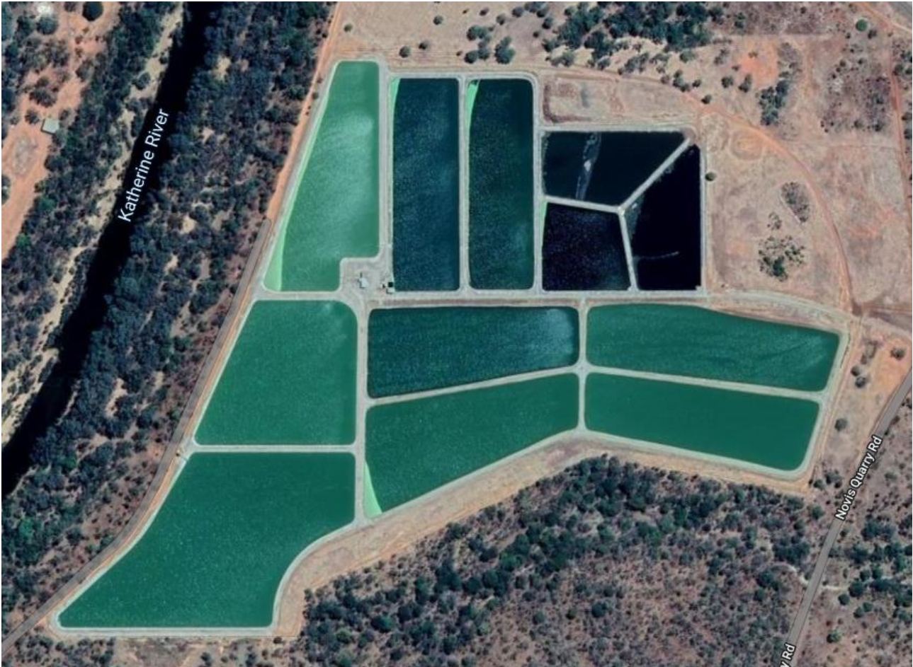
Figure 1: Katherine Waste Stabilisation Ponds (Google Image, 2022)
