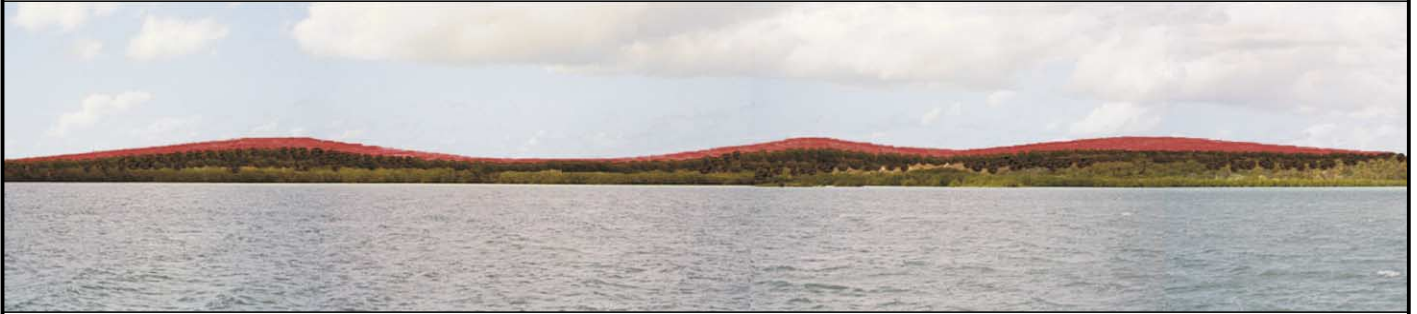
RDA AT FINAL HEIGHT WITH PROGRESSIVE REHABILITATION
