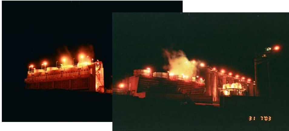
Photo 19 & 20. View from LM17 towards cooling towers and precipcs.
