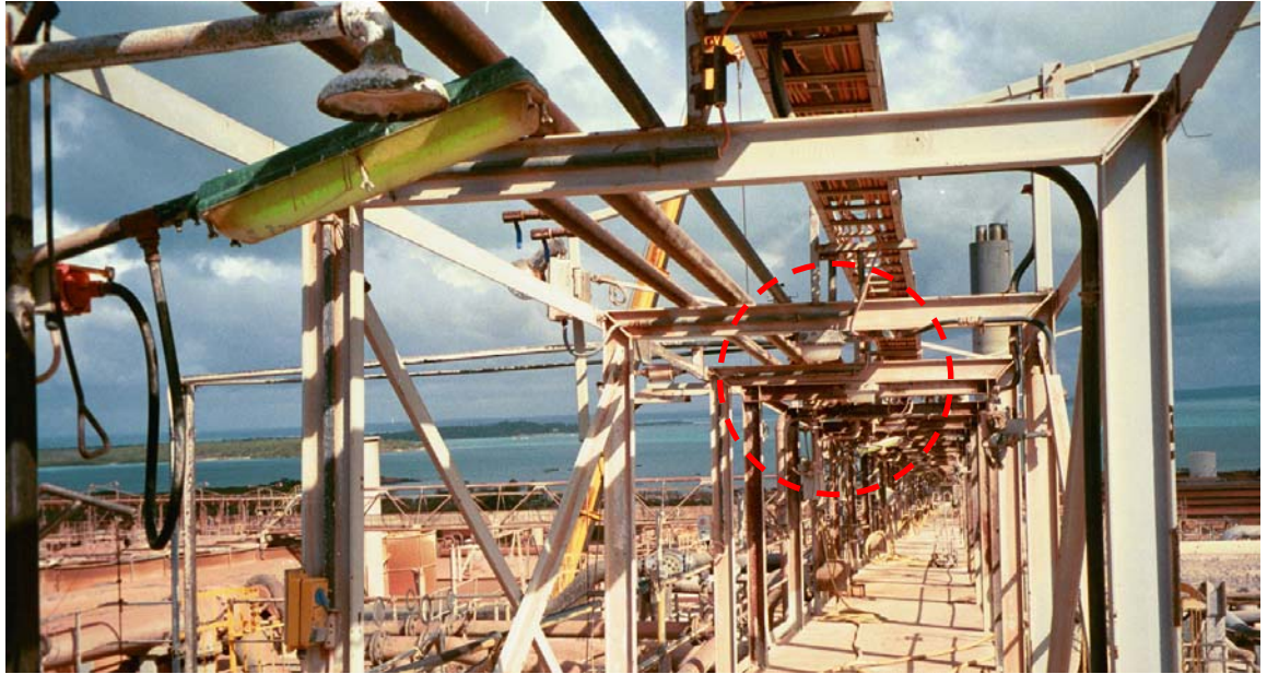
Photo 39. Bulkhead luminaires on high level walkways above precipitates.
