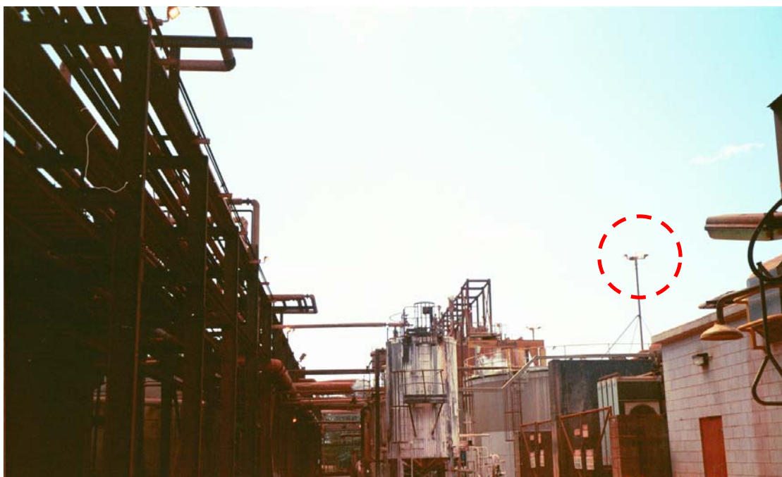
Photo 46. Azmet floodlights on pole above thickner tanks.
