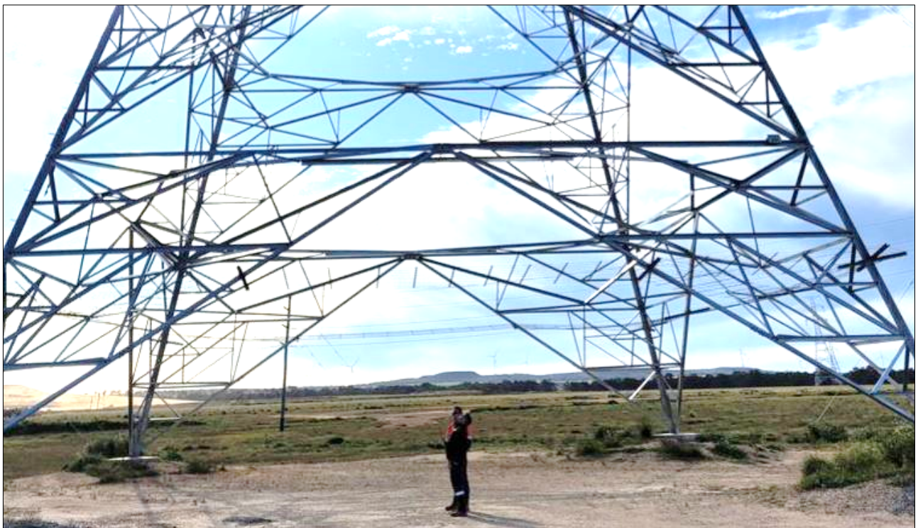
Figure 5. Photograph of an indicative tower pad
