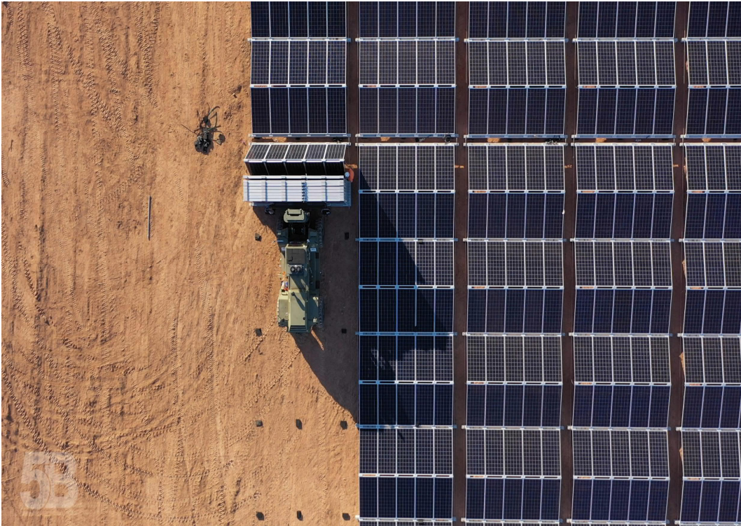
Figure 2-21. Deployment of a pre-fabricated MAV solar unit (Source: 5B, 2020)
