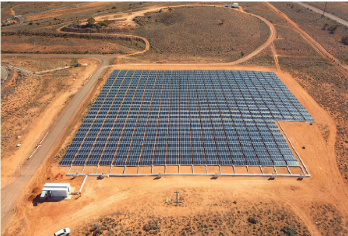
Figure 2-17. Example of a pre-fabricated (Maverick units) solar array, Port Bonython, SA (Source: 5B, 2020).
