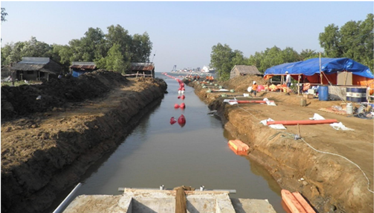
Figure 2-41. Photo example of open cut trench at landfall (Source: Sun Cable)
