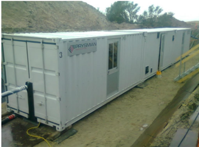
Figure 2-40. Photo of typical jointing containers (Source: Prysmian)
