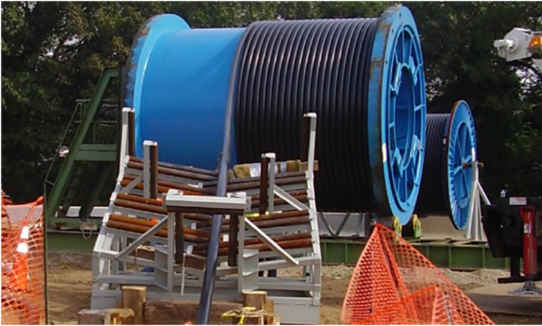
Figure 2-38. Photo example of motorised stand and roller placement used to install onshore cables (Source: Prysmian)
