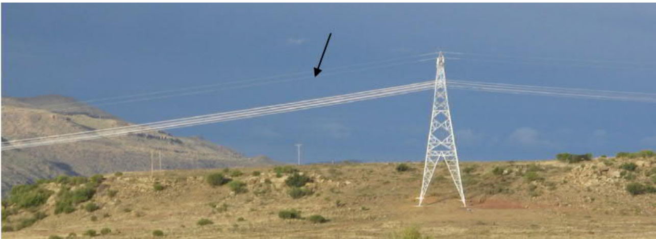
Figure 5-12. Photograph showing how hard it is to see powerline earth wires compared with conductors (from Prinsen et al. 2011)
